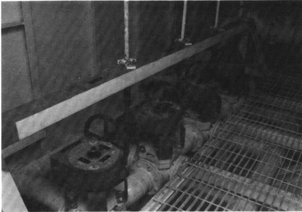
FIGURE 2-15 Pump Room Manifold
