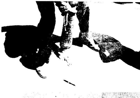
Forcing Hose onto Fitting
