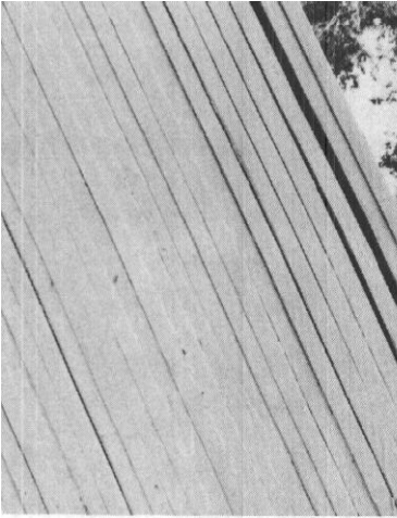
Figure 4-5. Glulam arches with rating 40. (A) Severe delamination in a localized area in the outer laminations.
