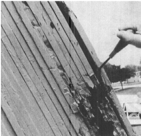
Figure 4-5. (C) Combination of delamination and severe decay. This condition was limited to the outer one-fifth of the member; any more extensive decay and delamination or any evidence of settlement should be rated as 20.
