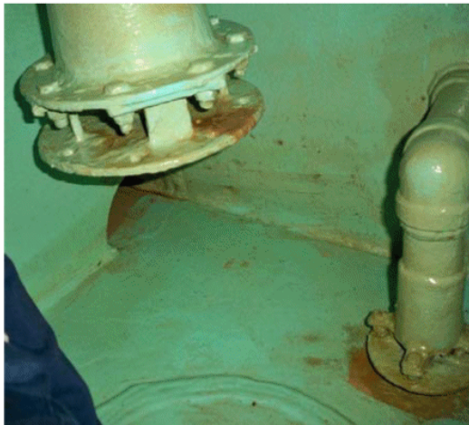
A. Waster Installed On Pipe
