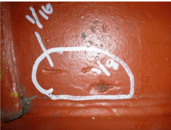
Gouges in Plate
