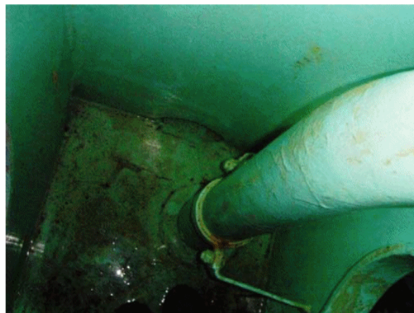
B. Waster (Doubler) Installed on Structure
