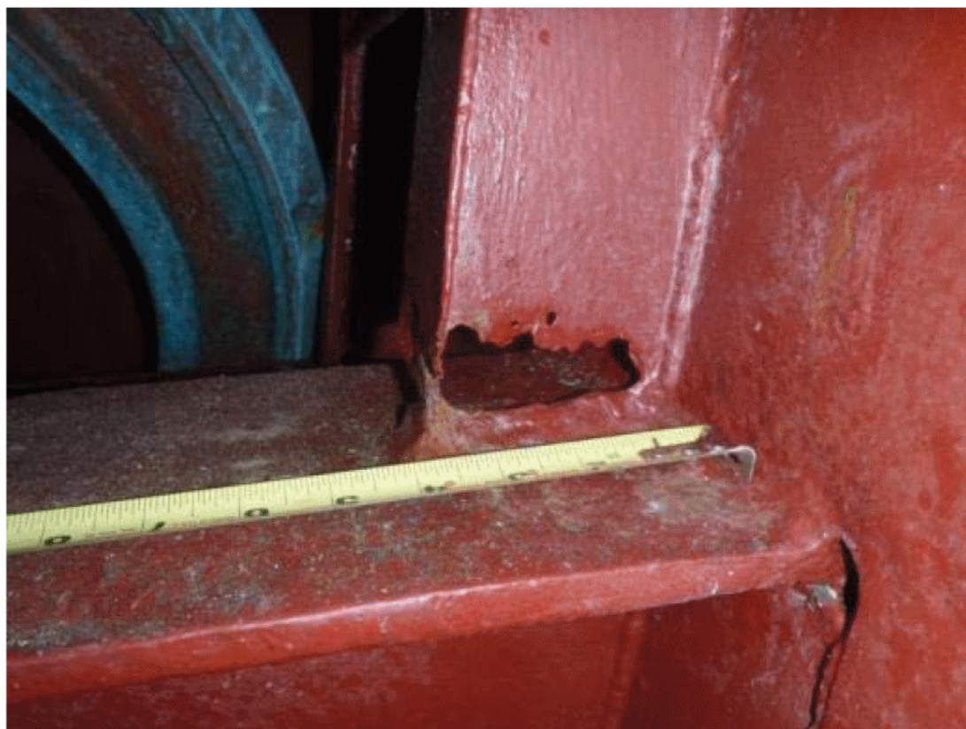
Holed and Painted Vertical Stiffener
