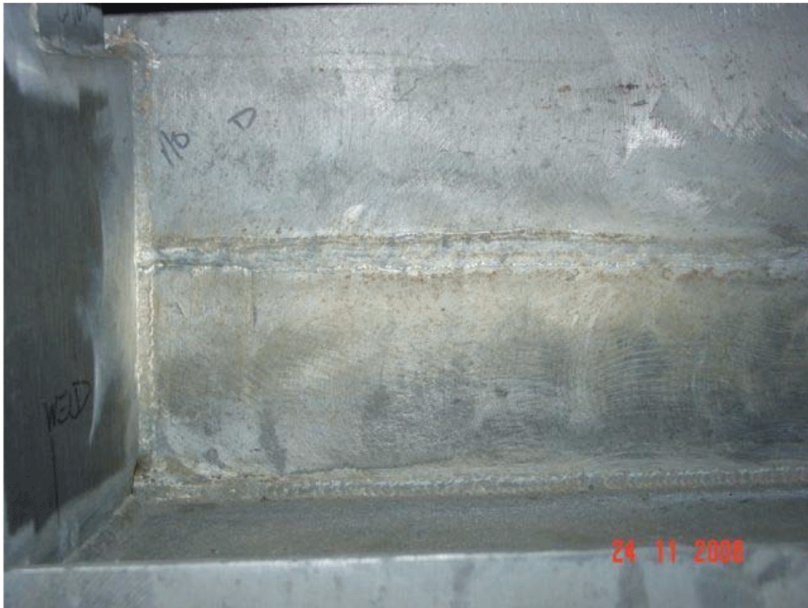
Figure 4-1 Bare Aluminum Water Tank With Acceptable Oxidation
