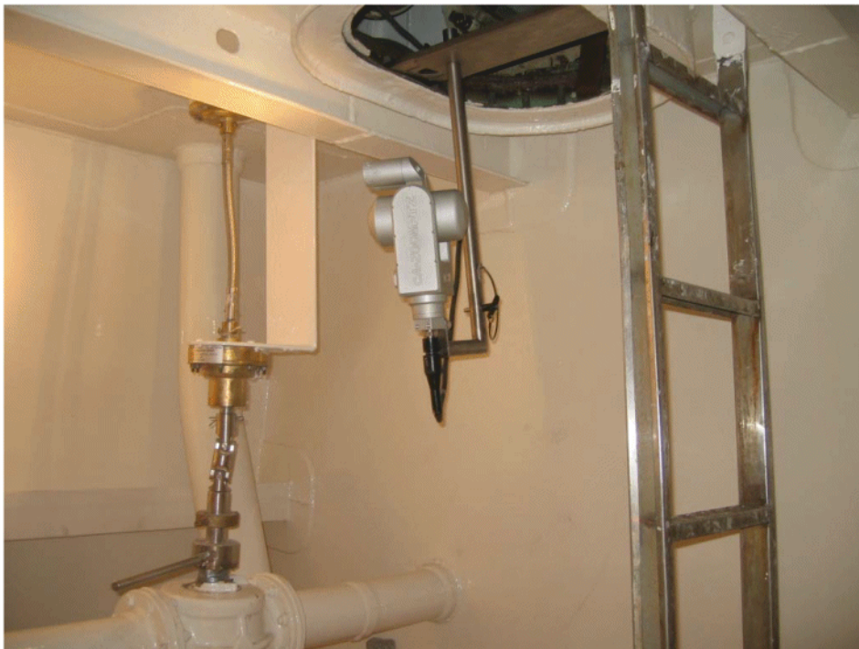
Figure 3-4 Example of ISIS Tank Assessment Without Human Entry
