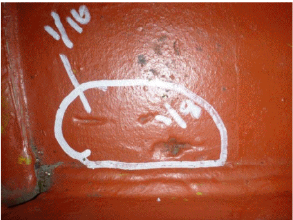
Gouges in Plate
