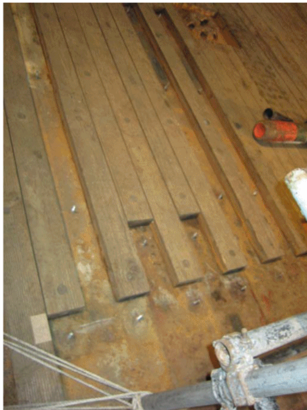
D. Well Deck Under Wood Beach Boards
