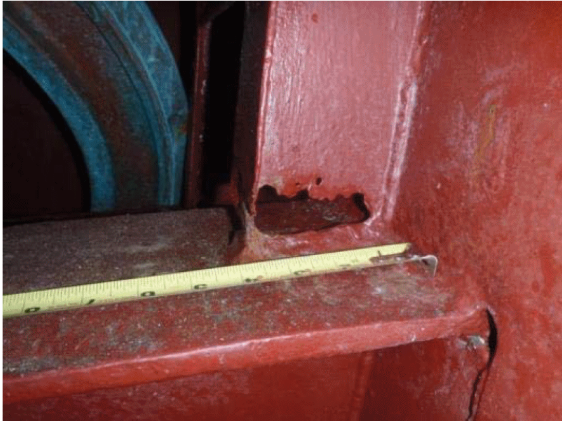
Holed and Painted Vertical Stiffener
