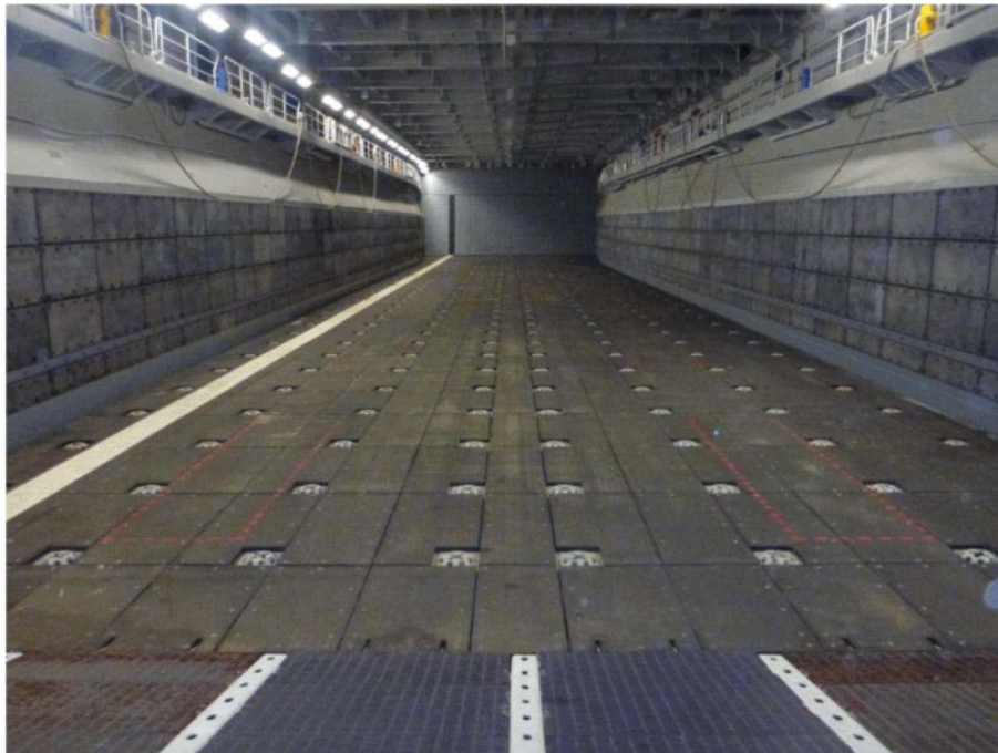
A. Composite Material Beach Boards and Batter Boards in Well Deck
