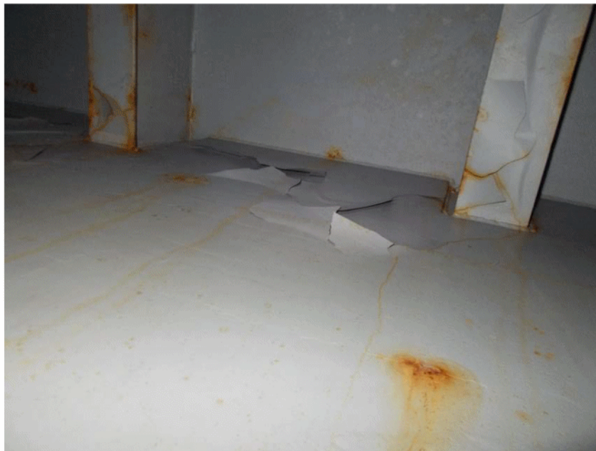
Delaminated Topcoat
