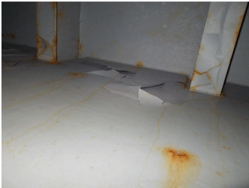
Delaminated Topcoat
