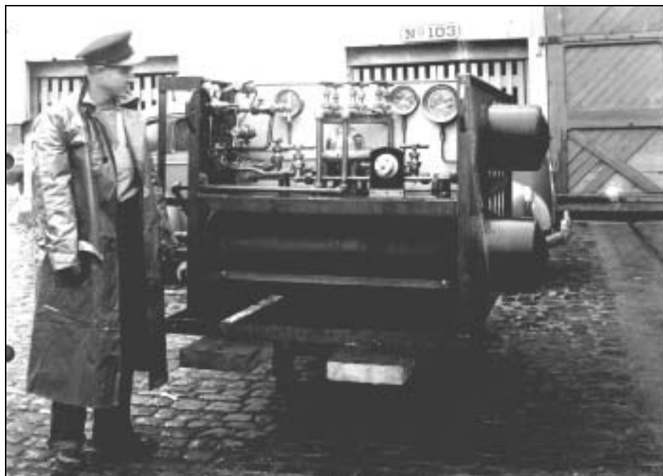
Figure 1-14. Helium-Oxygen Diving Manifold.
