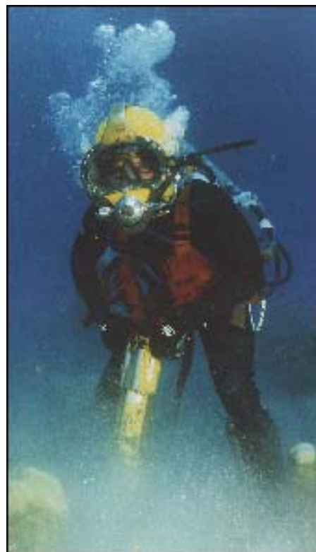
Figure 6-4. Underwater Construction Diving.
