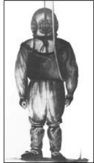
Figure 1-5. Siebe's First Enclosed Diving Dress and Helmet.
