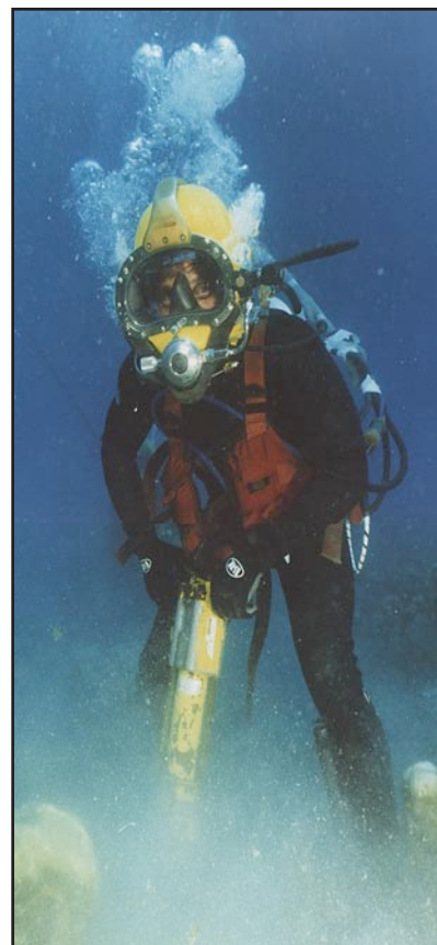
Figure 6-4. Underwater Construction Diving.
