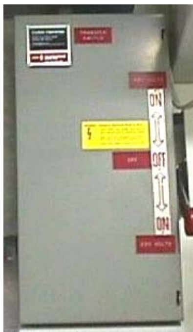
Figure 3-2. Manual Bus Transfer (MBT) Switch
