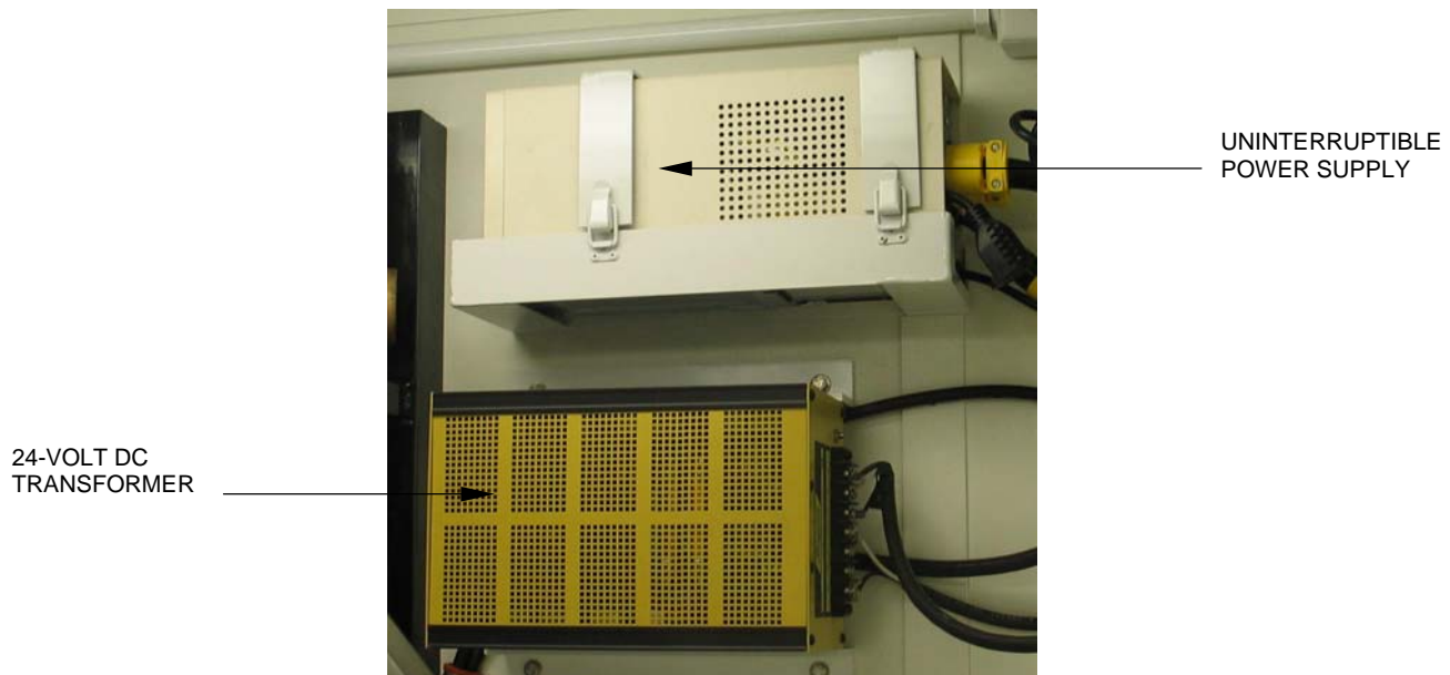
Figure 3-4. Uninterruptible Power Supply and Transformer
