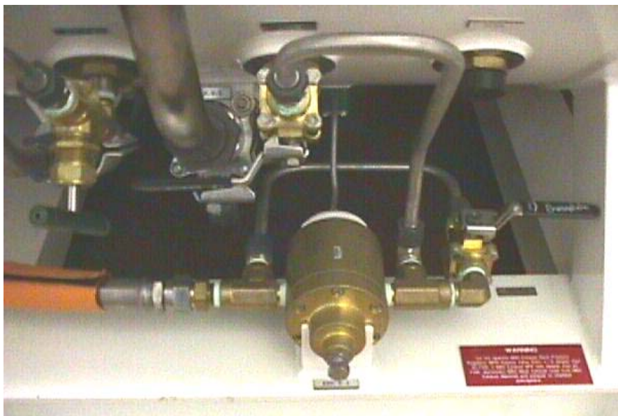
Figure 3-20. BIBS Exhaust Back Pressure Regulator
