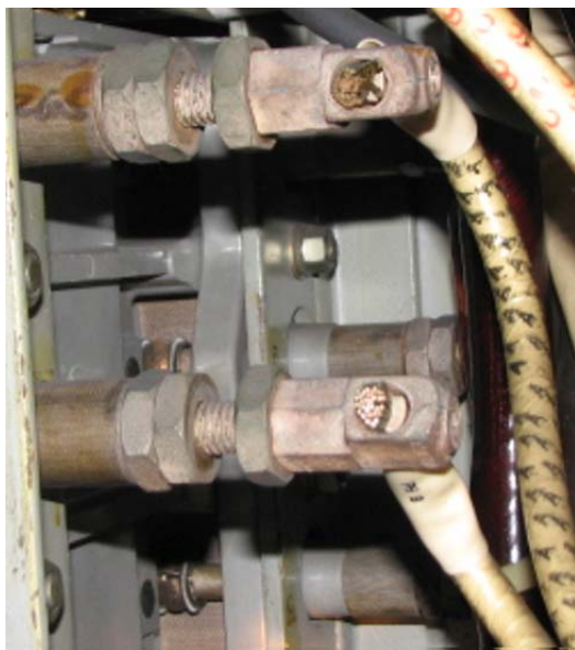
Figure 3-4. Two Possible Styles of Compression Type (DOSSERT) Cable Lug Connectors and Make-up to Circuit Breaker/Fuse Clip Current Stud
