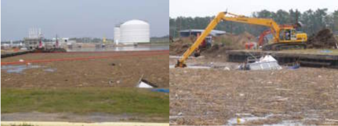
Figure 5-17. Debris removal in Lake Charles LNG turning basin.
