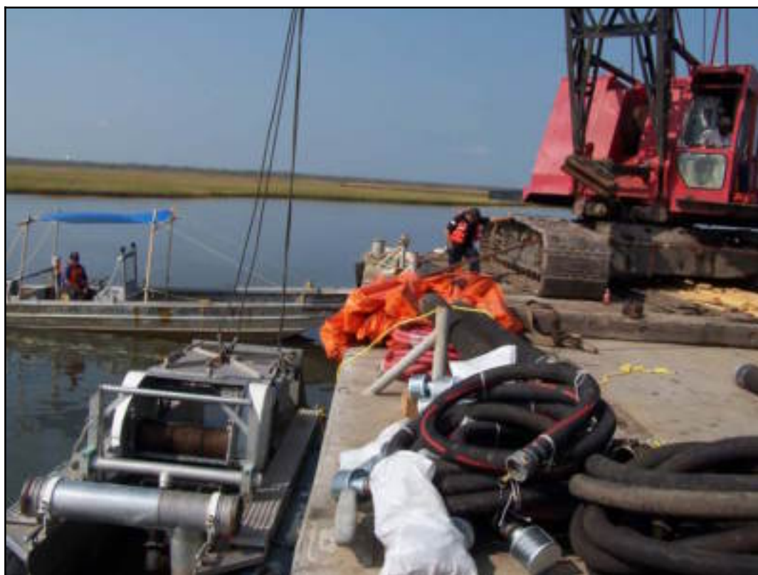
Figure H-8. Crane on Barge Launching the Skimmer
