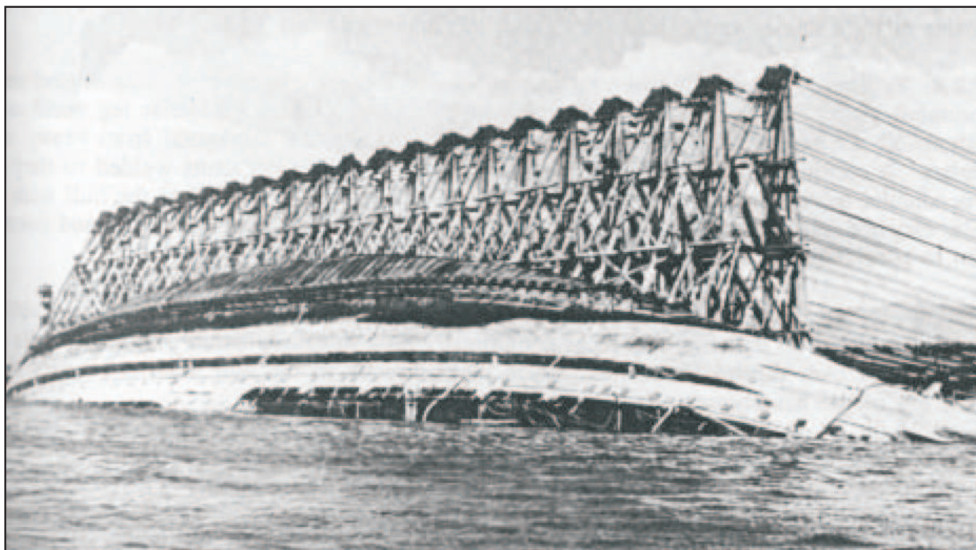
Figure 7-15. Braced-Girder Headframes on USS OKLAHOMA.
