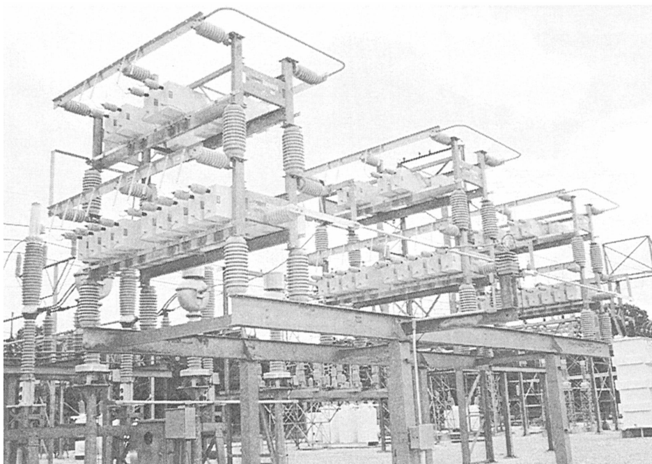
Figure 4-29.—Capacitors, open-rack installation.
