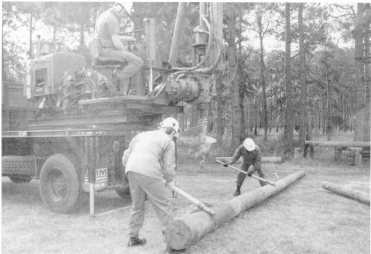
Figure 4-51.—Pole positioning before being set.
