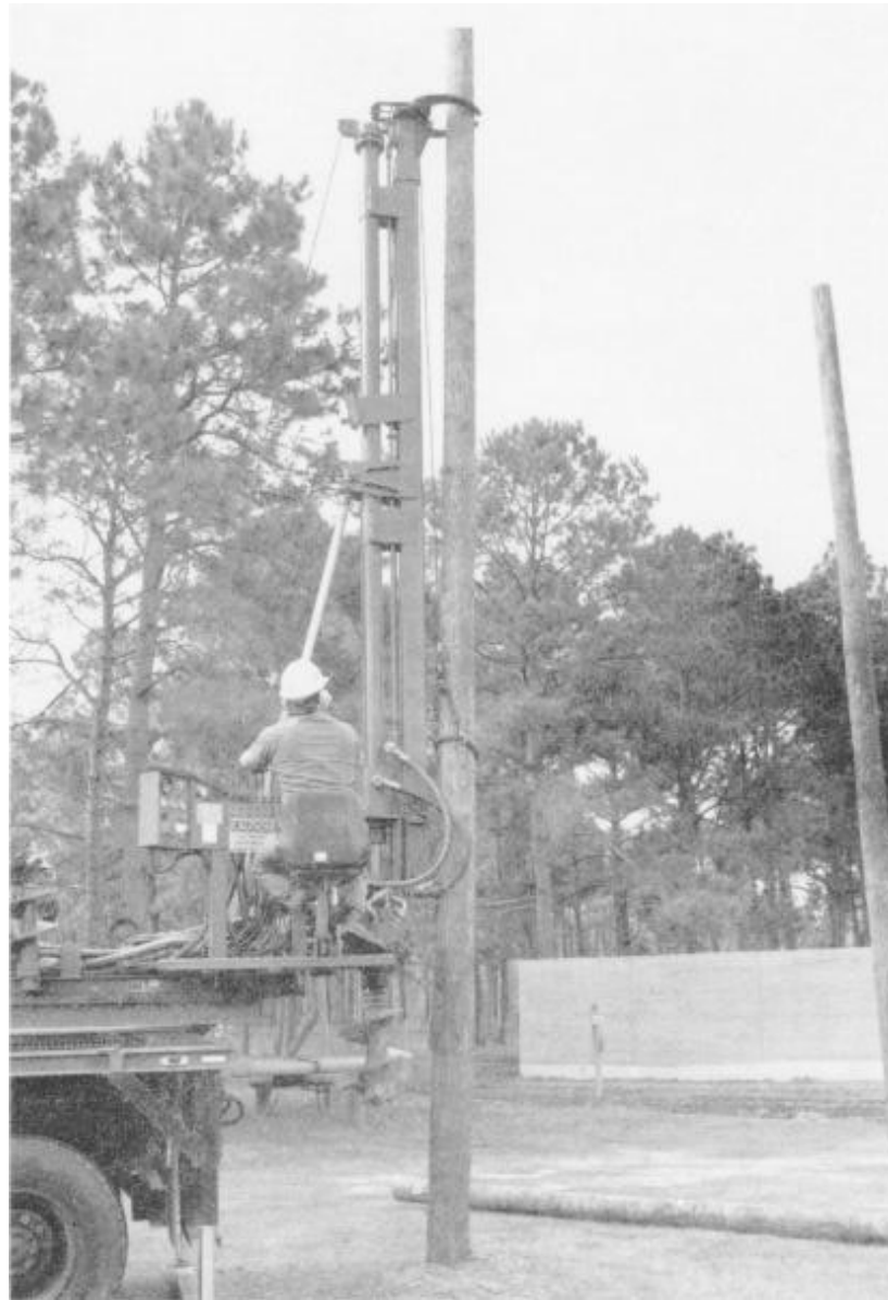
Figure 4-52.—Auger truck setting a pole.
