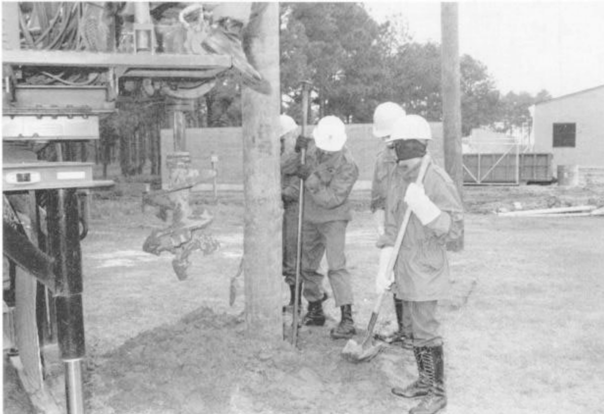
Figure 4-58.—Tamping and backfilling erected pole.
