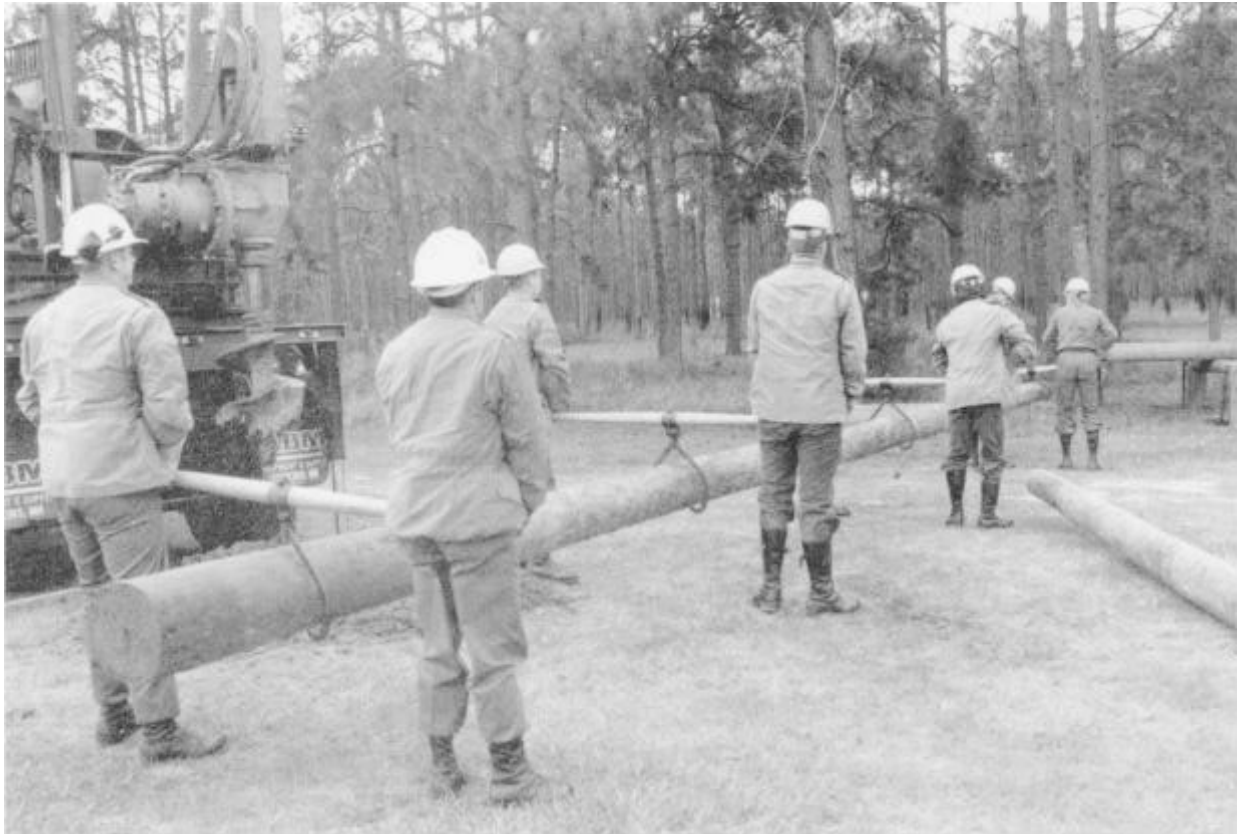
Figure 4-54.—Manually positioning a pole.
