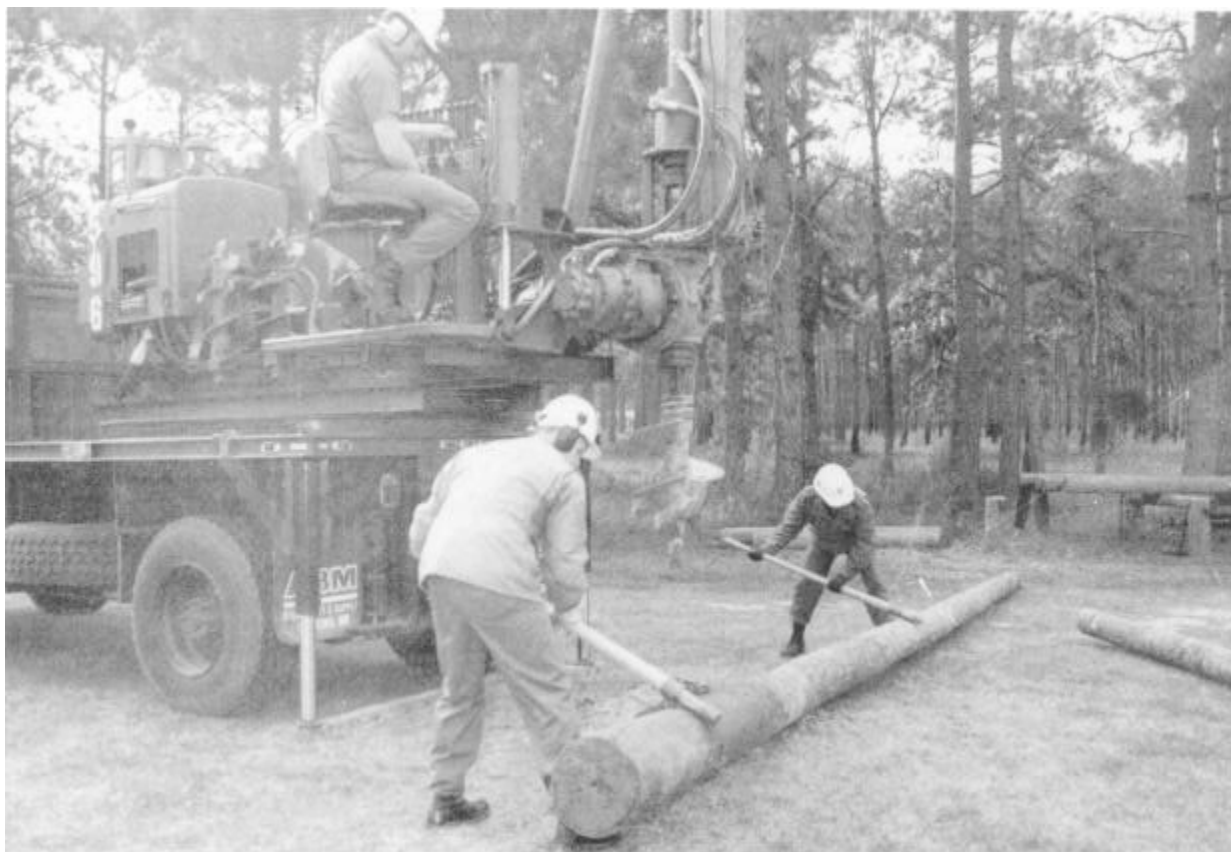
Figure 4-51.—Pole positioning before being set.
