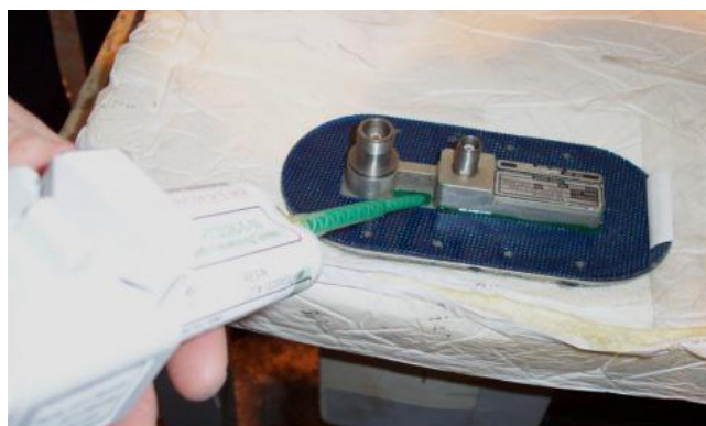
Figure 6-4. Application of Self-Leveling Green Sealant
