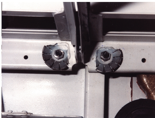
Figure 6-5. EMI Bonding Washers in Avionics Bay
