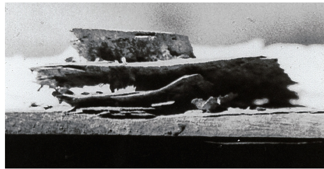
Figure 3-14. Extreme Example of Exfoliation at Edge of Sheet
