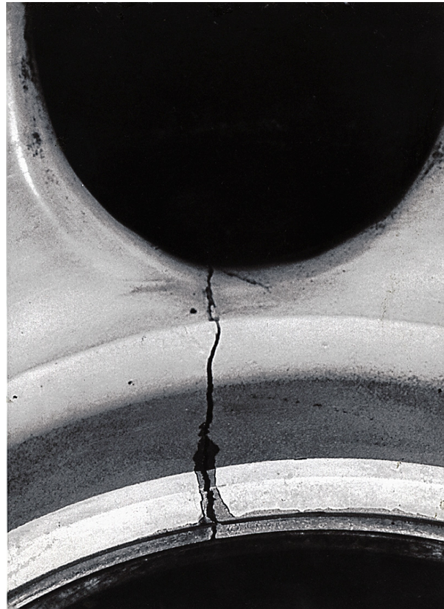
Figure 3-19. Cracking (Typical of Stress Corrosion or Corrosion Fatigue)
