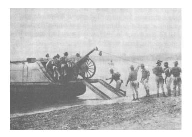
"In the early 1920s, the Marines experimented with a British-designed 'Beetle boat' and a Christie amphibian tractor. . . . In 1936, the Marines tried out five different commercial boats as possible landing craft. They even tested fishing boats and boats seized from rum runners; but all had exposed rudders and propellers, and men had to drop as far as 10 feet into the water.
