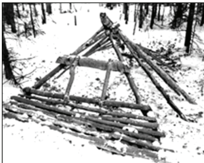
Figure 2-1. Frame of infrared counterdetection (thermal) shelter
