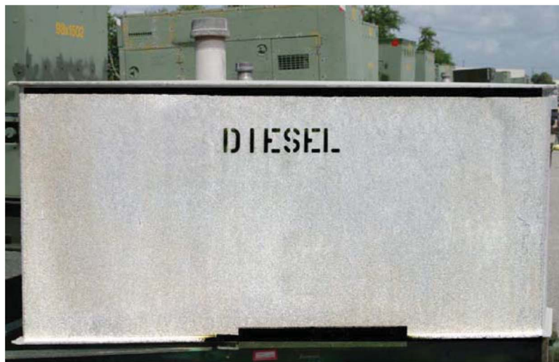
Figure 1-6. Example of Uniform Etch
