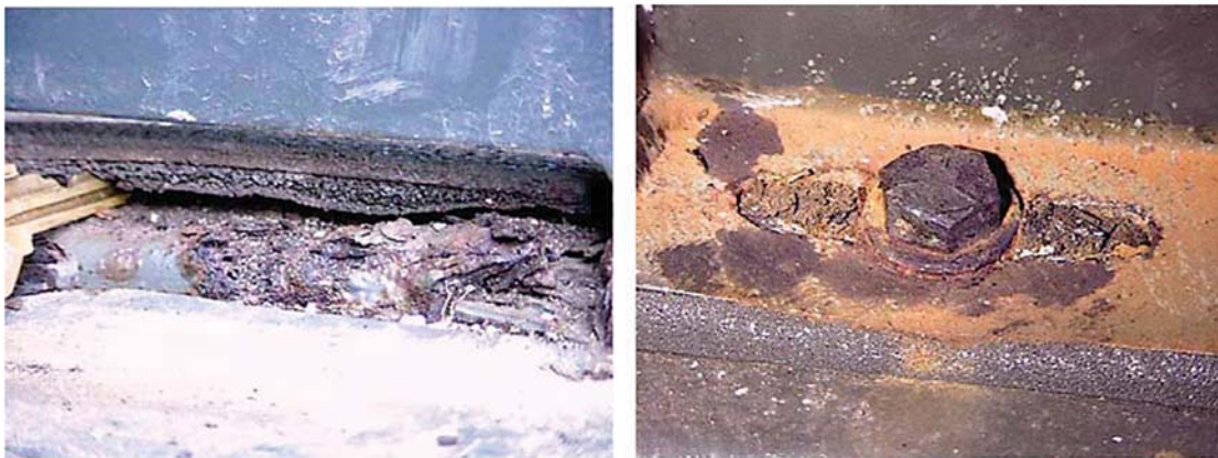
Figure 1-4. Open Cell Foam and Resulting Corrosion
