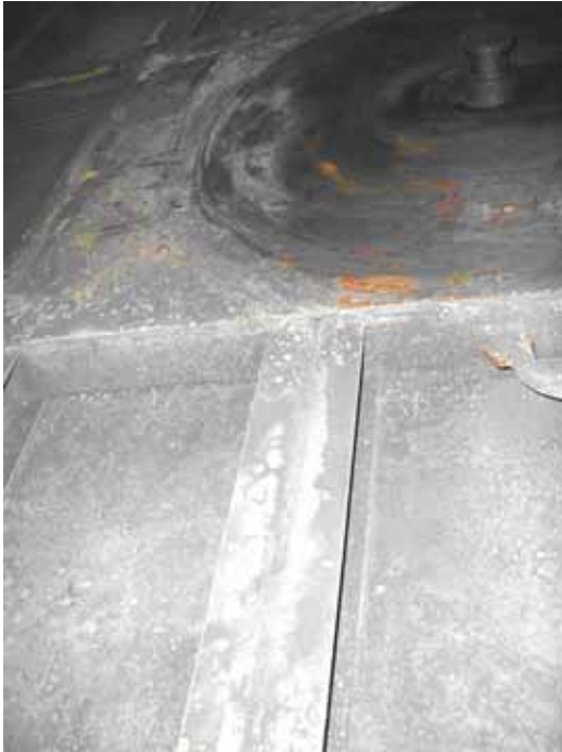
Figure 10-13. Corrosion Undercarriage of Shelter
