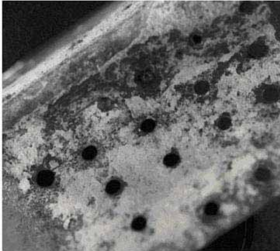
Figure 3-20. Aluminum Surface Corrosion Products
