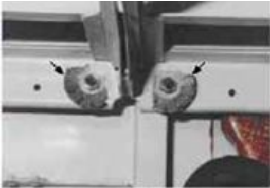
Figure 10-15. EMI Bonding Washers for Electronics
