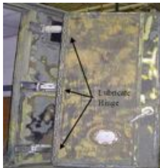
Figure 10-8. Electronic Shelter Door
