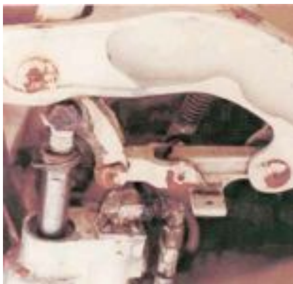
Figure 3-19. Steel Corrosion Products (Rust)
