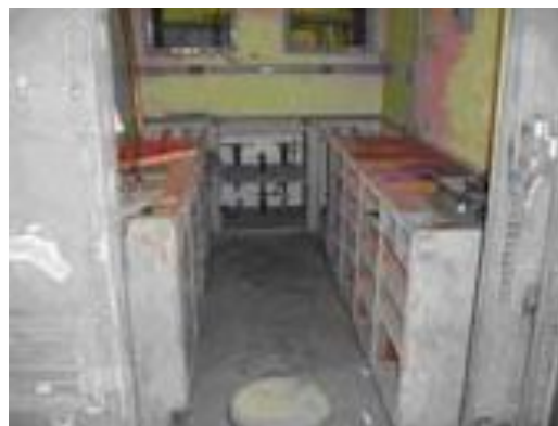
Figure 4-1. Electronic Shelter: Installed Wood Cabinetry
