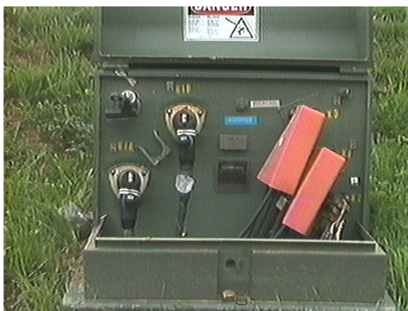
Picture 2-3 Liquid-filled compartmentalized padmount transformer
