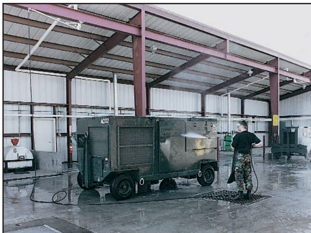
An exterior, semi-enclosed wash rack.
