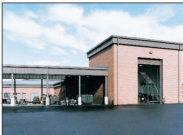
High bay access is required for oversized equipment.
