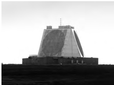
Figure 19-7. Solid state PAR at Fylingdales. (Royal Air Force photo)
