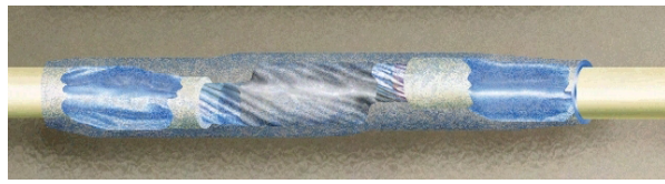
Figure 19-13. Fully Melted Solder Sleeve
