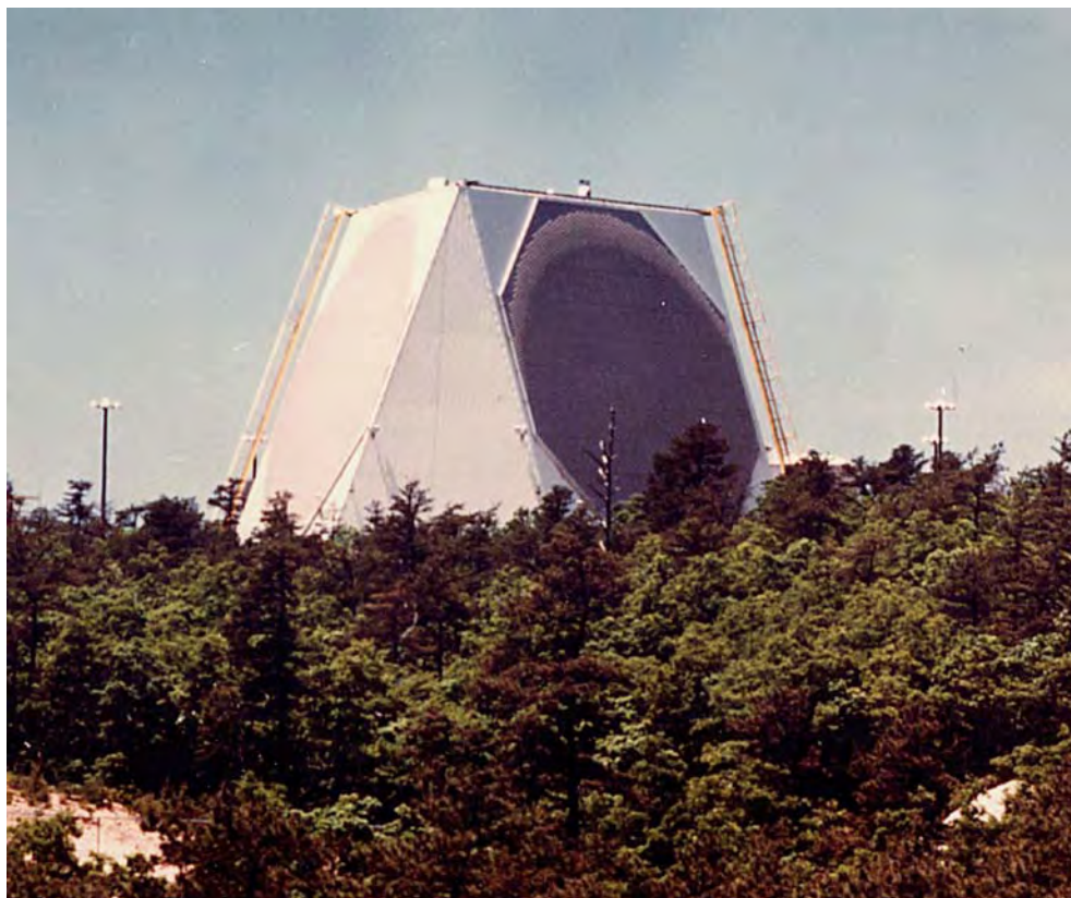
Figure 4.4-5. PAVE PAWS 2-sided phased-array radar.
