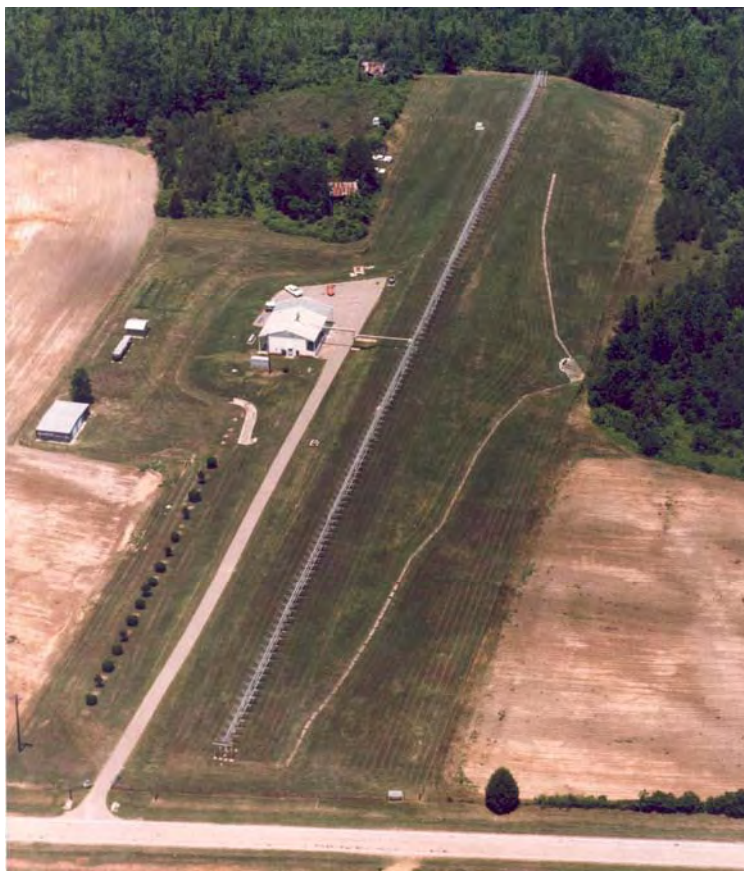
Figure 4.4-11. Jordan Lake transmitter of the USAF Space Surveillance Fence near Wetumpka, Alabama.
