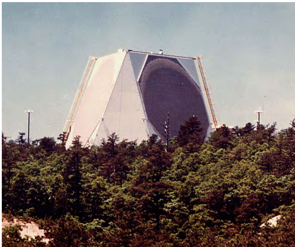
Figure 4.4-5. PAVE PAWS 2-sided phased-array radar.
