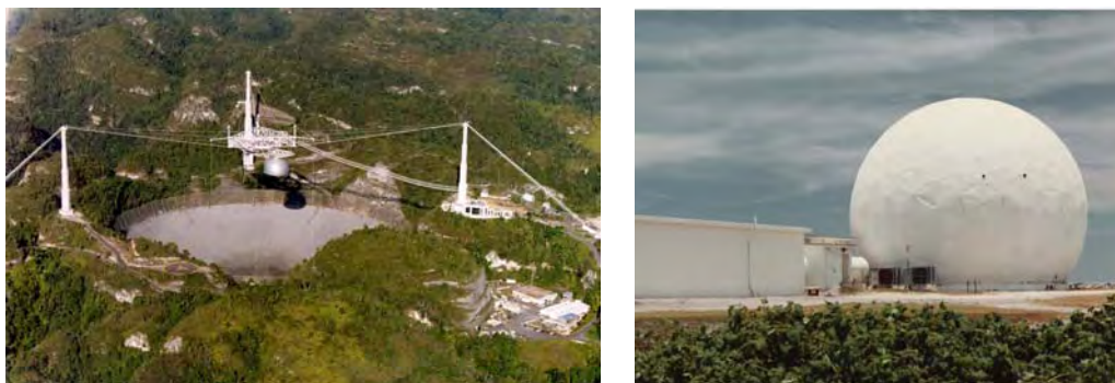
Figure 4.4-16. Arecibo and ALCOR antennas.
