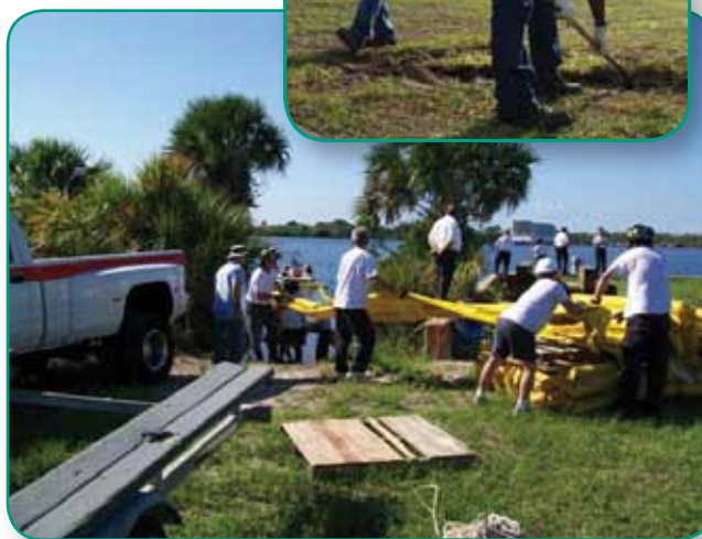
Post Emergency Response Cleanup Team practices deploying booms to prevent spill migration within the Turn Basin.
