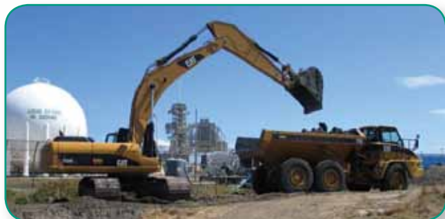
Excavation activities in the Launch Pad 39A area resulted in removal of a contaminated source area.
