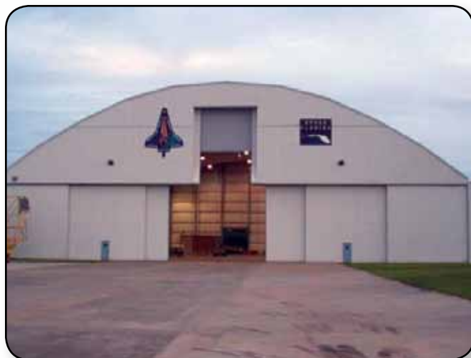
A view of the main hangar door of the Reusable Launch Vehicle Hangar.
