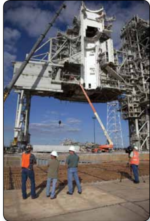
The rotating service structure on Launch Pad 39B is being dismantled at Kennedy Space Center.
