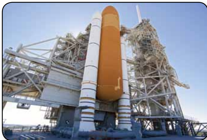
Space shuttle Discovery's external tank and solid rocket boosters are seen in this view of Launch Pad 39A at Kennedy Space Center. To the right is the fixed service structure and to the left is the rotating service structure.
