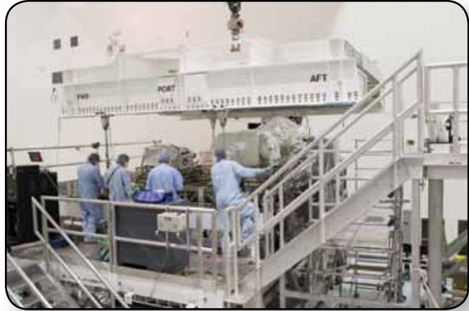
A technician in the Space Station Processing Facility measures the weight and center of gravity of the EXPRESS Logistics Carrier-1 (ELC-1).
