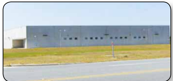
A view of the Utility Shop Facility located in Kennedy Space Center's Launch Complex 39 Area.
