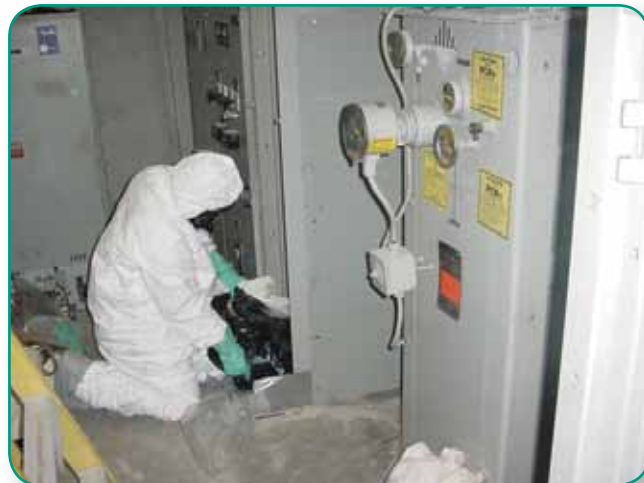
A technician removes contaminated oil from a Kennedy Space Center transformer.
