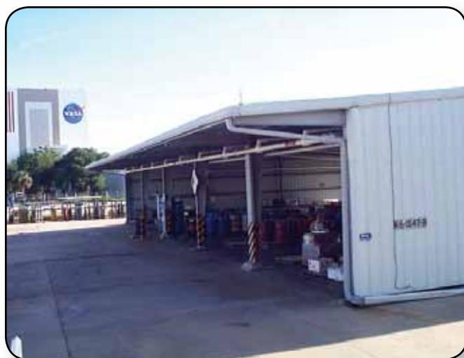
The Barrel Shed supports a number of activities associated with the Logistics Facility.
