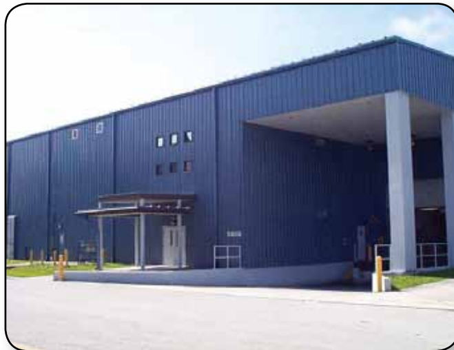
Assembly and Refurbishment Facility Storage Building loading dock area.
