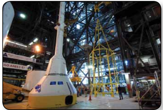
In the Vehicle Assembly Building, the yellow framework at center is about to undergo a fit check. Nicknamed the "birdcage," it is the lifting fixture utilized to lift the Orion crew exploration vehicle and launch abort system.
