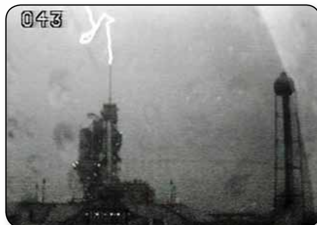
The lightning protection system protects the space shuttle Endeavour as lightning strikes the launch pad at Kennedy Space Center.
