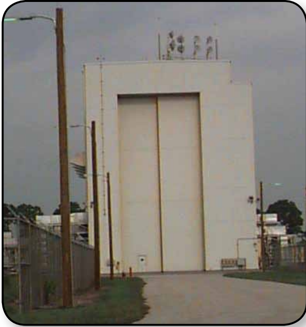
A view of the high bay door entrance into the Payload Hazardous Servicing Facility (PHSF).
