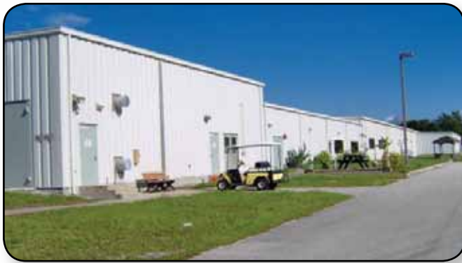
A view of the Multi-Operations Support Building in Kennedy Space Center's Industrial Area.
