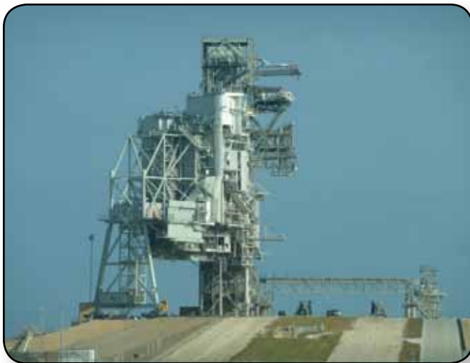
A view of Launch Pad 39B before work began to reconfigure it to support a "clean pad" concept. This concept supports a versatile system capable of launching a number of vehicles.
