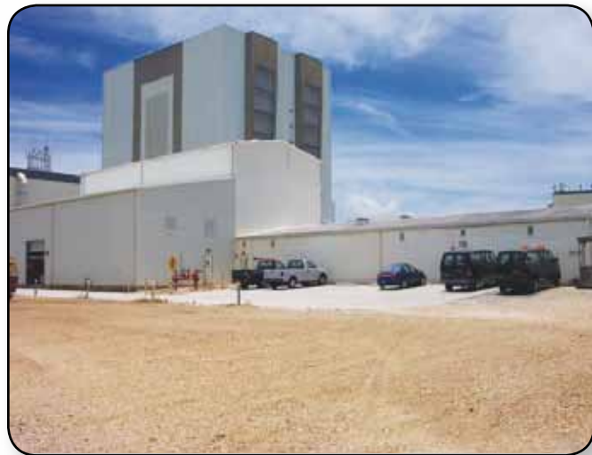
The Crawler Transporter Maintenance Facility.
