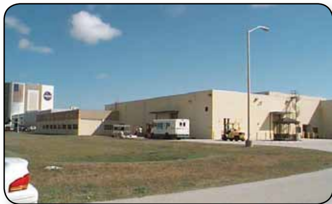
A view of the main entrance to the Component Refurbishment and Chemical Analysis Facility.
