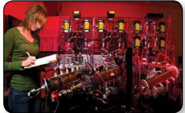
Kennedy Space Center's wastewater bioreactors purify wastewater by utilizing fiber membranes and microbial communities that convert ammonium nitrogen (e.g., from urine) into nitrate, or N 2 gas.
