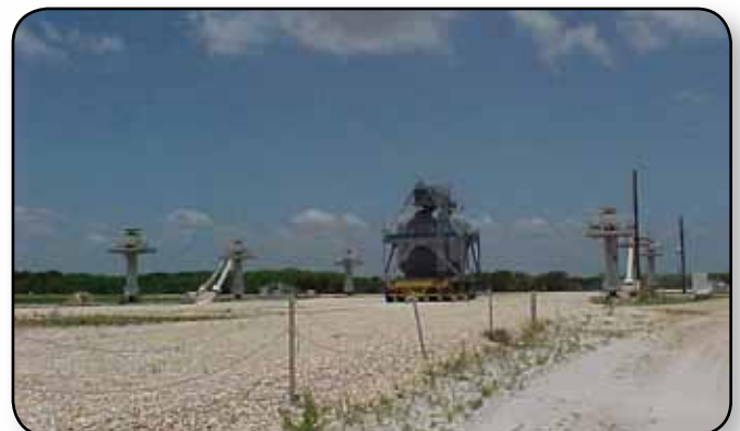
In the construction and refurbishment area at Kennedy Space Center, support pedestals are used for mobile launcher servicing.
