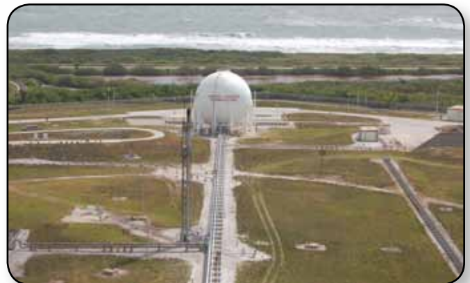
The 850,000-gallon liquid hydrogen tank, pictured here, and the 900,000-gallon liquid oxygen tank and cryogenic supply systems support Kennedy Space Center's Launch Complex 39.
