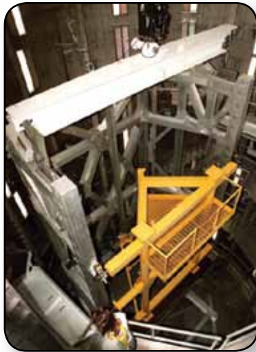
In the Operations and Checkout Building's high bay, the Rotation Handling Fixture (RHF), with a simulated module attached, is viewed from above the altitude chamber into which it was lowered during a test.
