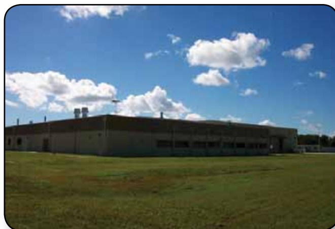
A view of the Component Refurbishment and Chemical Analysis Facility.
