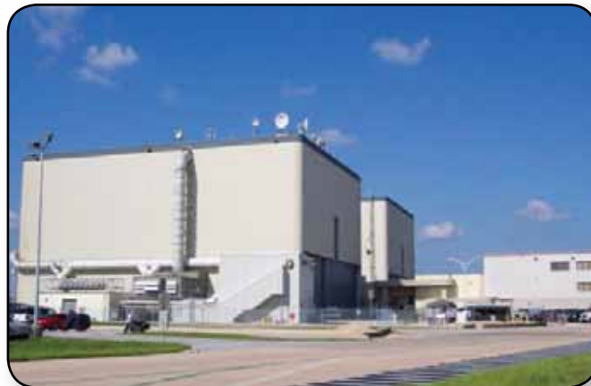
A view of Orbiter Processing Facilities 1 and 2. OPF 1 is in the foreground.
