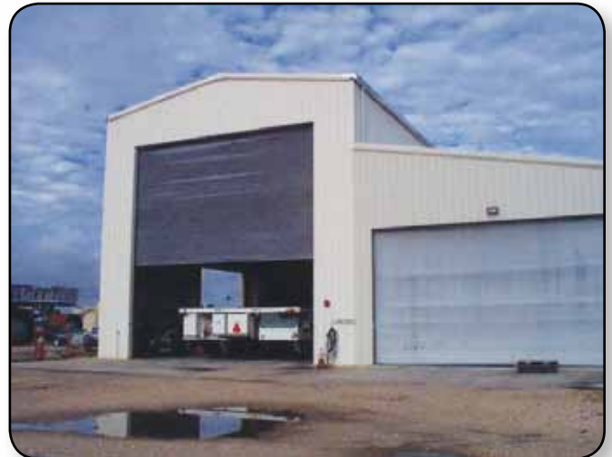
The Crawler Transporter Maintenance Facility.
