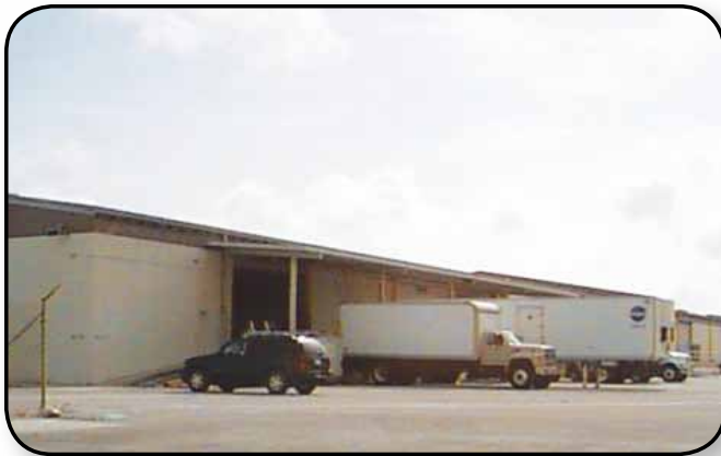
A view of the loading dock area of Supply Warehouse No. 1 at Kennedy Space Center in Florida.
