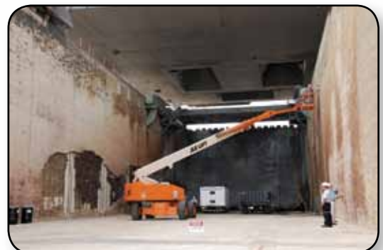
A view of the flame trench on Launch Pad 39A at Kennedy Space Center, shows where damage occurred during launch of space shuttle Discovery on the STS-124 mission, May 31, 2008.
