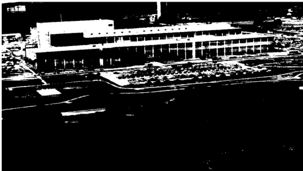
Figure 2-1. Operations and Checkout (O&C) Building
