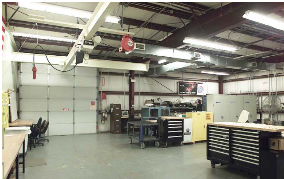
Figure 20. Building 993 High Bay Work Area
