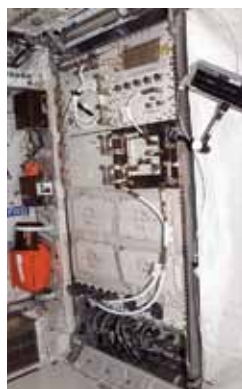
Provides sub-rack-sized experiments with standard utilities such as power, data, and cooling.
