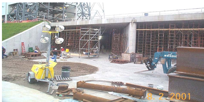
Figure 53:- Ripple effect repair work being accomplished at Launch Complex 37
