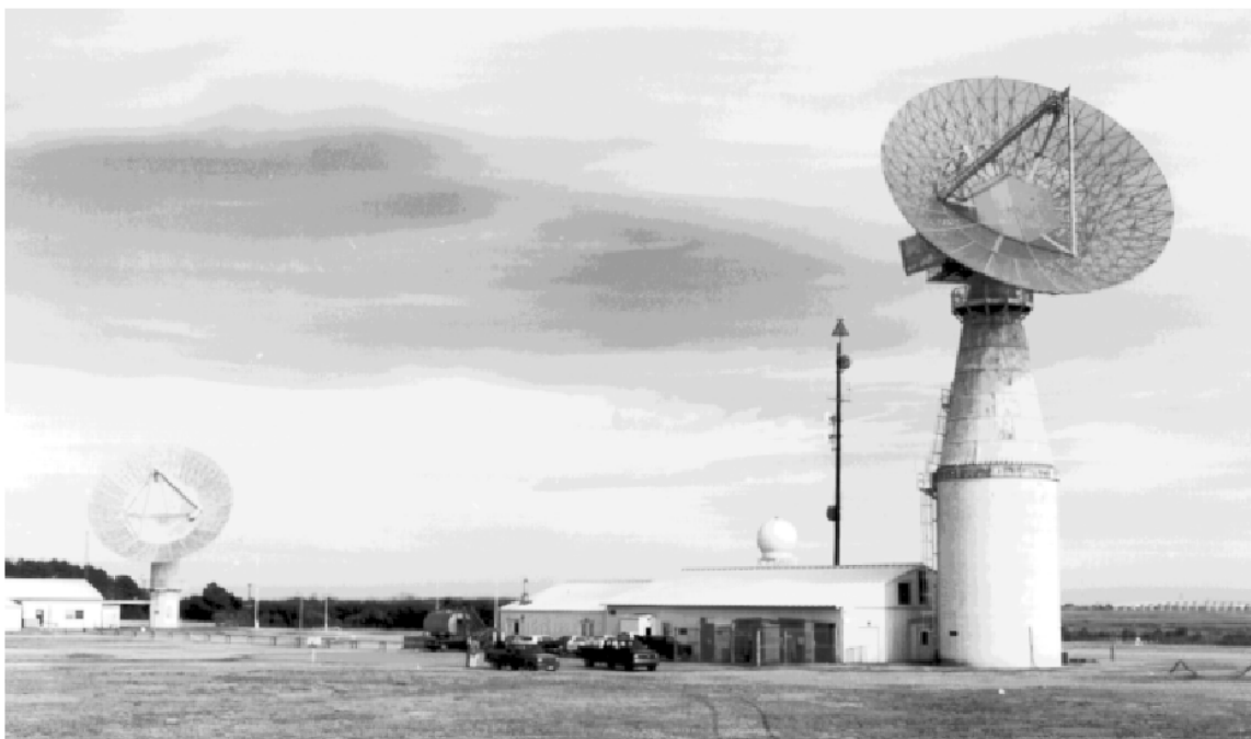
Figure 3-30. Atmospheric Sciences Research Facility
