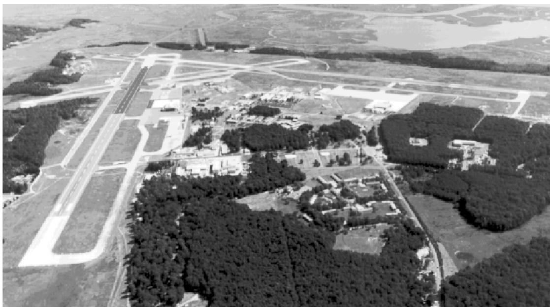
Figure 3-1. Aerial View of the Wallops Main Base
