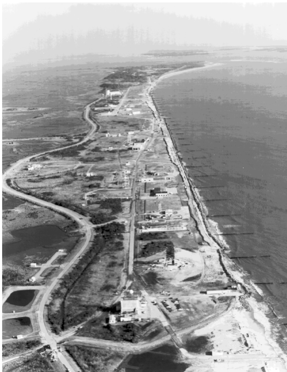
Figure 3-3. Aerial View of Wallops Island
