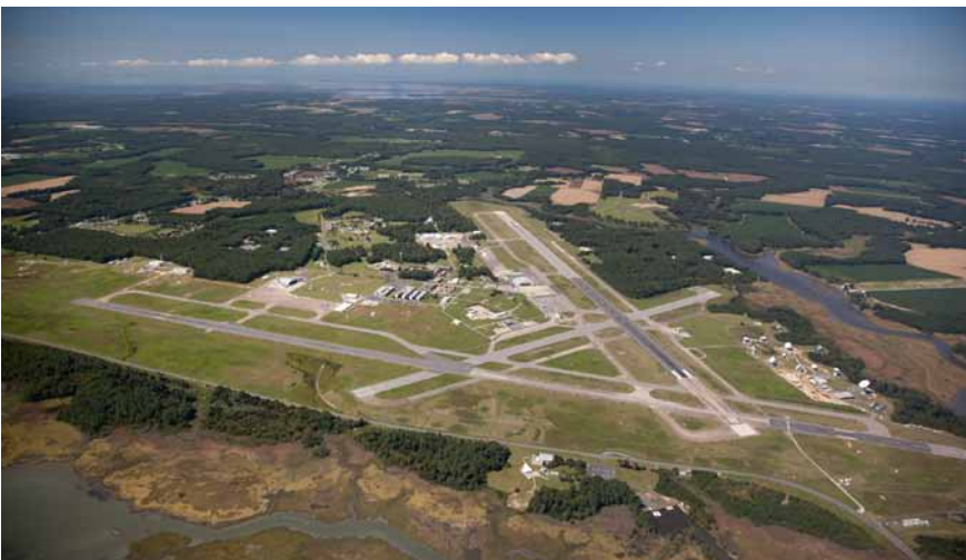
Figure 3-1. Aerial View of the Wallops Main Base
