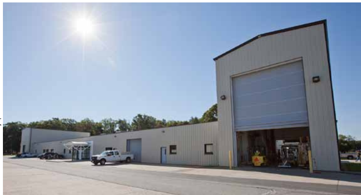
Figure 3-15. Multi-Payload Processing Facility (MPPF)
