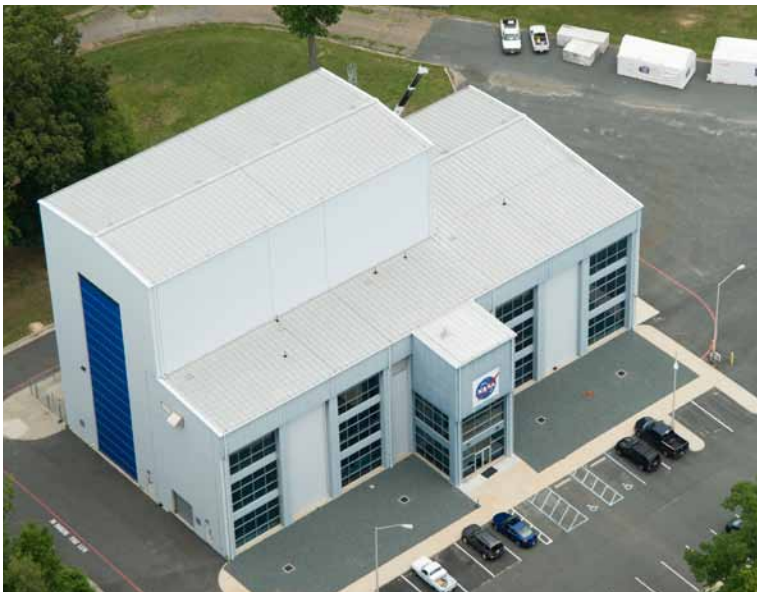
Figure 3-10. H-100 Payload Processing Facility (PPF)
