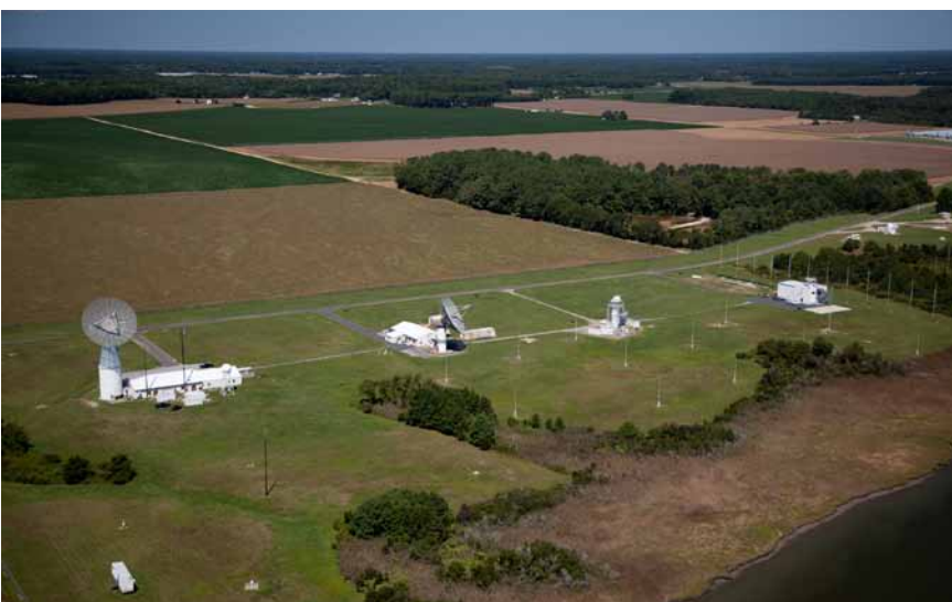
Figure 3-2. Aerial View of the Wallops Mainland
