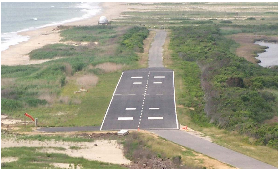
Figure 5. UAV Runway on Wallops Island
