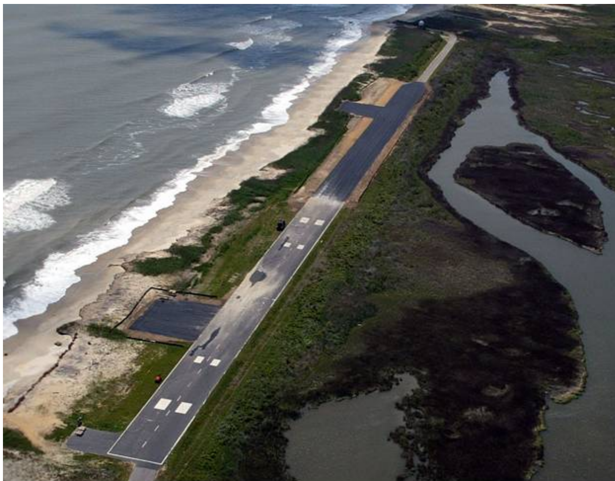
Figure 8. UAV Runway on Wallops Island
