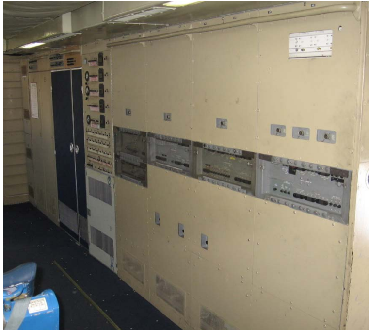
Figure 4-14. Electrical load center
