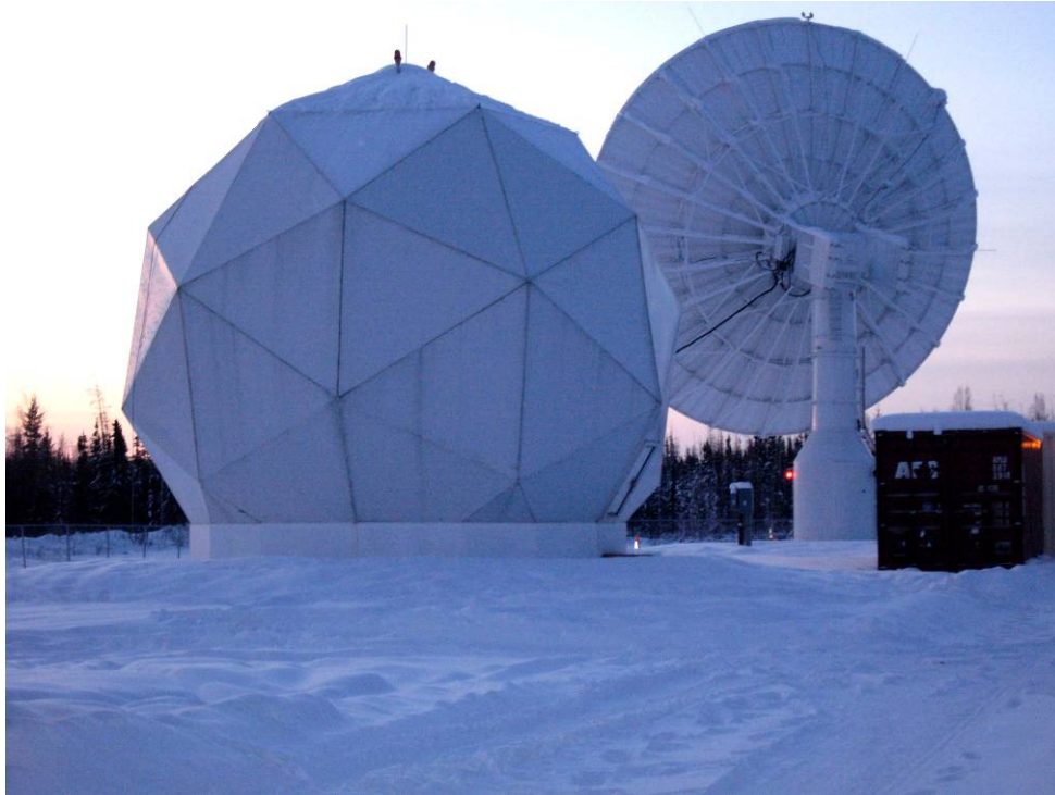
Figure 6-4. North Pole ground station. (USA-K02 in foreground within radome, USA-K01 in background)
