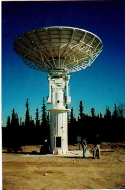
Figure 6-2a. PF2 Antenna Before Radome Installation
