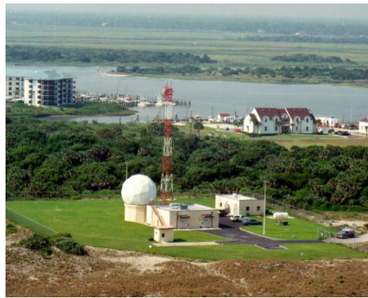
Figure 8-2. PDL Ground Station
