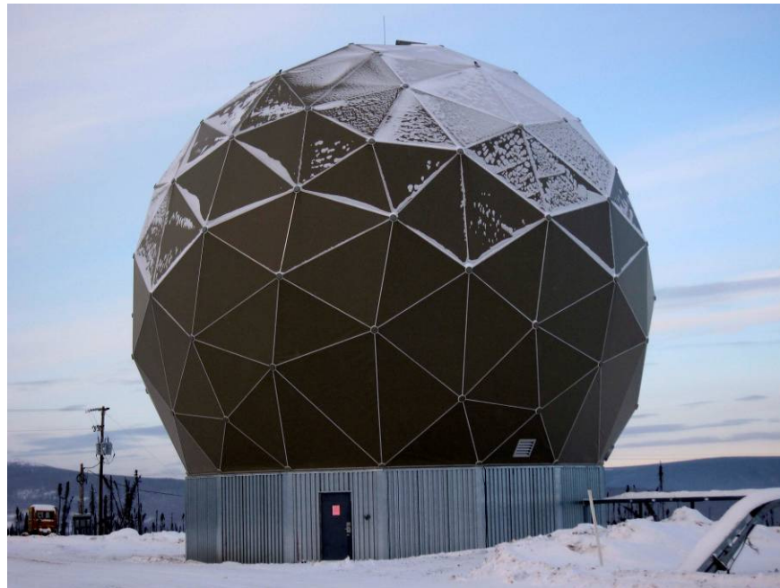
Figure 6-2. PF2 Antenna Radome
