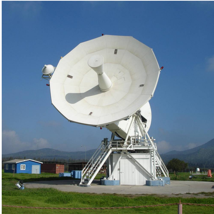
Figure 10-1 AGO 9-m Antenna
