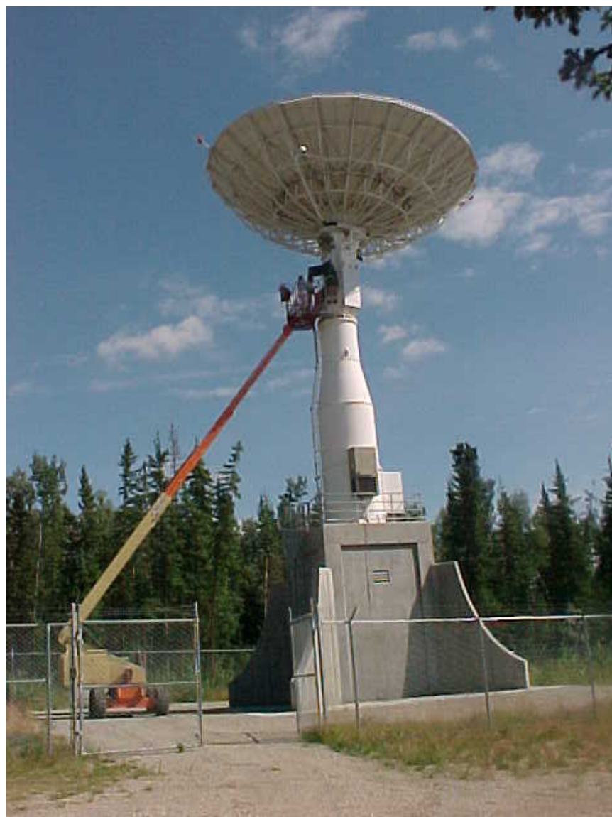
Figure 7-2. ASF 11-Meter Antenna
