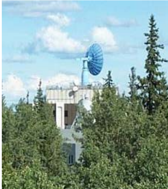
Figure 7-1. ASF 10-meter Antenna
