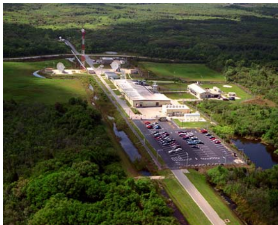
Figure 8-1. MILA Ground Station
