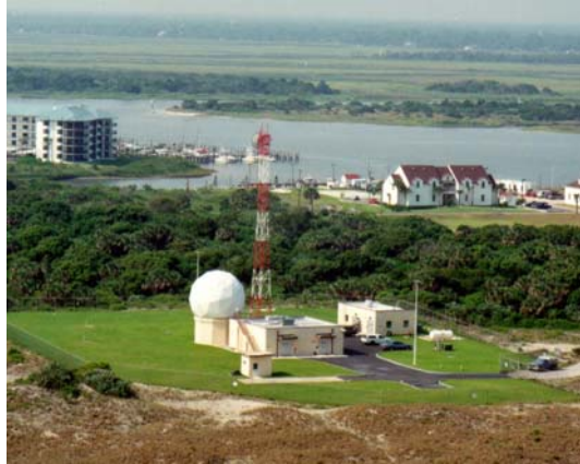
Figure 8-2. PDL Ground Station
