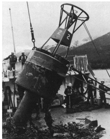
Figure 509. Buoy showing counterweight.
