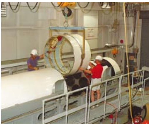
Figure 3-30: An interstage being positioned for attachment.
