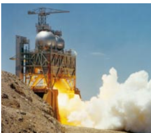
Figure 15-13: A single liquid rocket engine vertical test stand.
