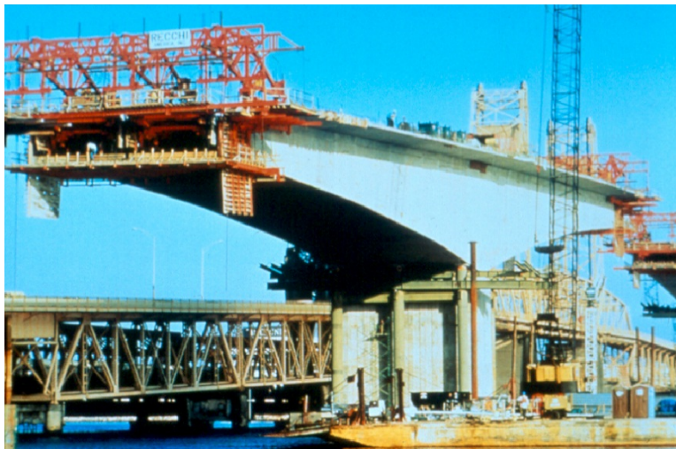
Figure 1.17 - Cast-In-Place Segmental Construction using Form Travelers
