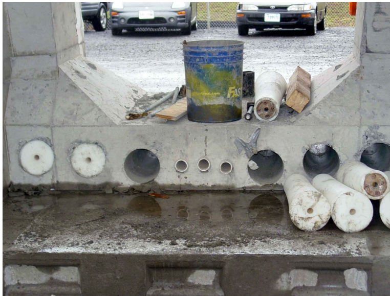
Figure 2.12 - Reusable Diabolo Inserts at Deviation Segment
