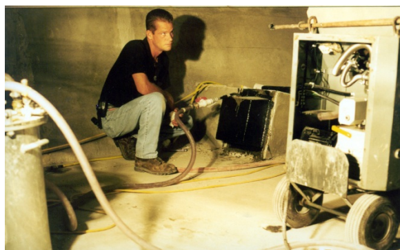
Figure 4.2 - Vacuum Grouting Equipment, Digital Volumeter (up (upper left), Void Volume Measurement (upper right), Grout Pump (lower left), Vacuum Grout injection (lower right)
