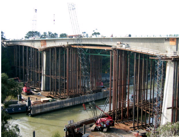
Figure 1.6 - Cast-In-Place Post-Tensioned Construction in California
