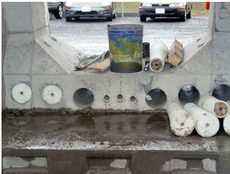
Figure 2.12 - Reusable Diabolo Inserts at Deviation Segment
