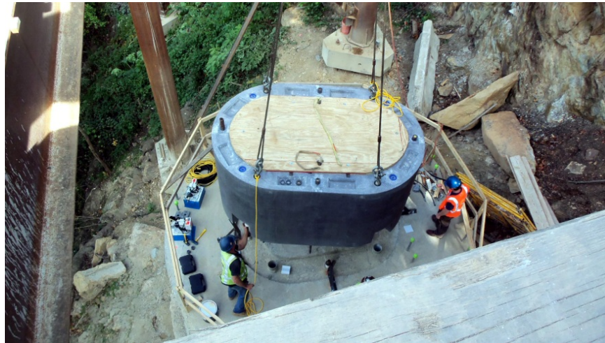
Figure 1.32 - Precast Hollow Segmental Piers, Foothills Bridge No. 2
