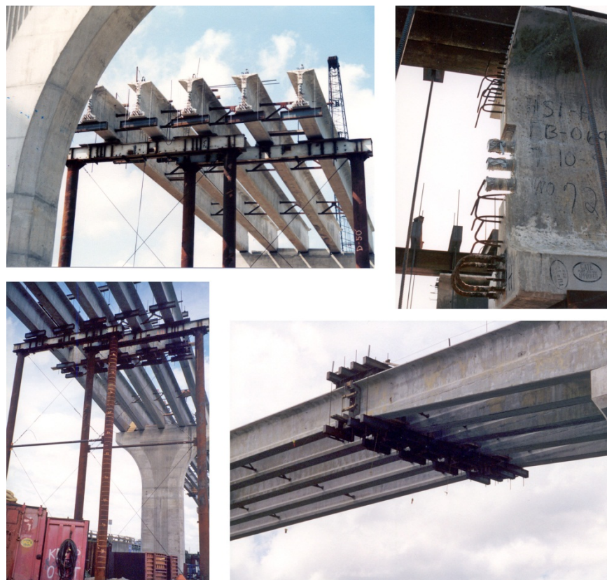
Figure 1.7 - Spliced Haunched I-Girder of Main Span Unit
