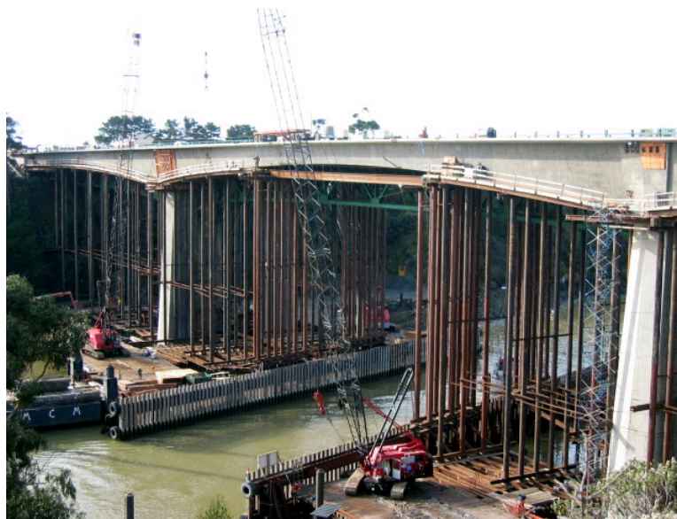
Figure 1.6 - Cast-In-Place Post-Tensioned Construction in California
