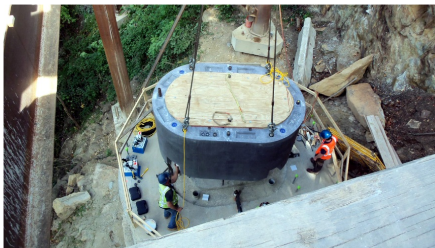
Figure 1.32 - Precast Hollow Segmental Piers, Foothills Bridge No. 2
