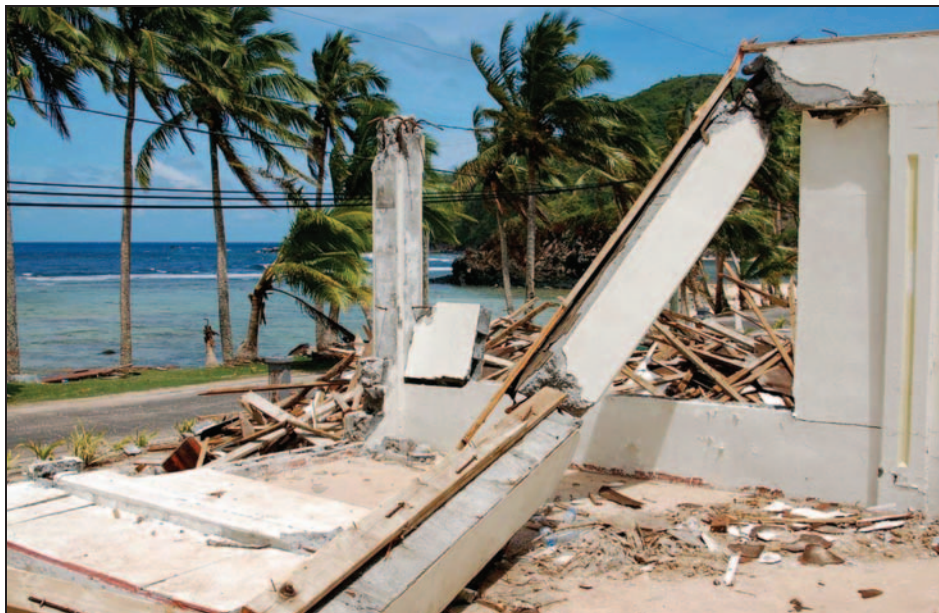
Figure 3-12. Damage from the 2009 tsunami (Amanave, American Samoa)
