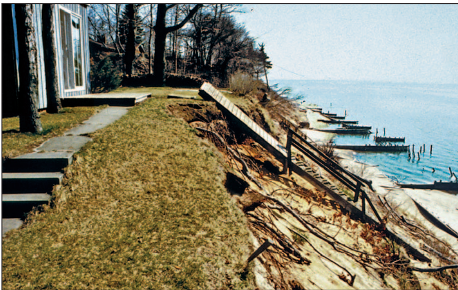
Figure 2-7. Erosion along the Lake Michigan shoreline at Holland, MI, resulting from high lake levels and storm activity (August 1988)
