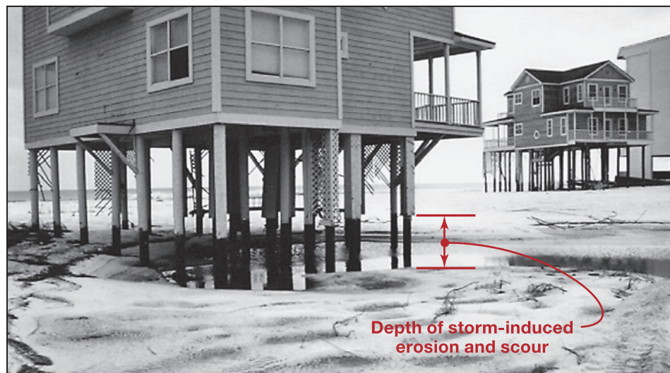
Figure 3-21. Pile-supported house in the area of channeled flow shown in Figure 3-20. The building foundation and elevation successfully prevented high-velocity flow, erosion, and scour from destroying this building
