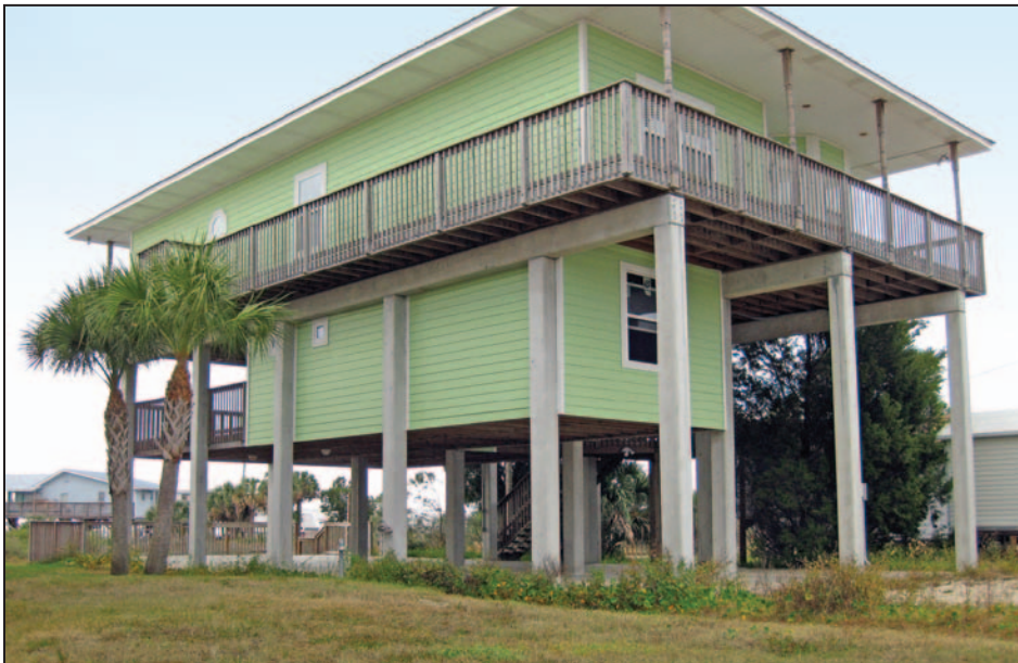
Figure 2-23. Above-grade enclosure (Perry, FL)
