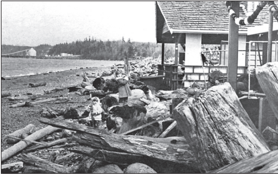
Figure 3-30. Drift logs driven into coastal houses at Sandy Point, WA, during a March 1975 storm
