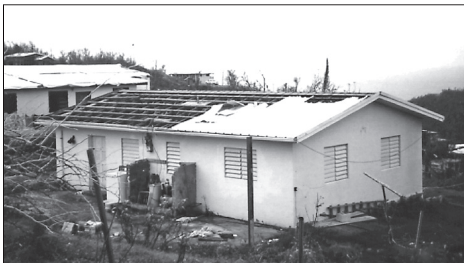
Figure 2-6. This house lost most of its metal roof covering due to high winds during Hurricane Marilyn in 1995 (location unknown) SOURCE: NRCA 1996
