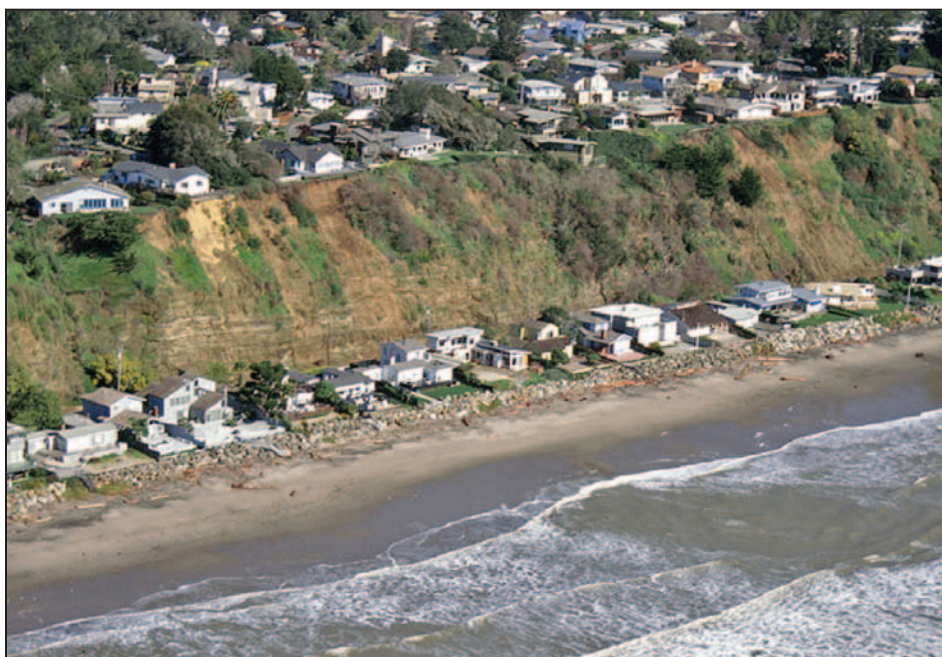
Figure 4-22. Coastal building site in Aptos, CA, provides an example of a coastal building site subject to multiple hazards
