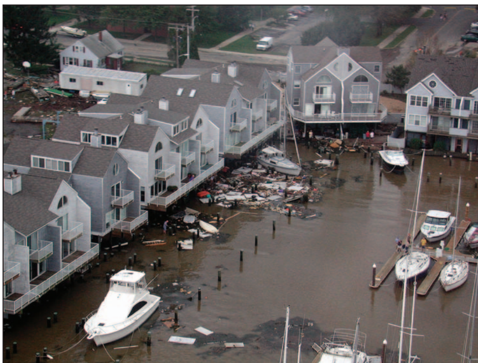
Figure 4-21. Condominiums built along the shoreline at the mouth of the Susquehanna River on the Chesapeake Bay were subjected to flood-borne debris after Hurricane Isabel (Havre de Grace, MD, 2003)
