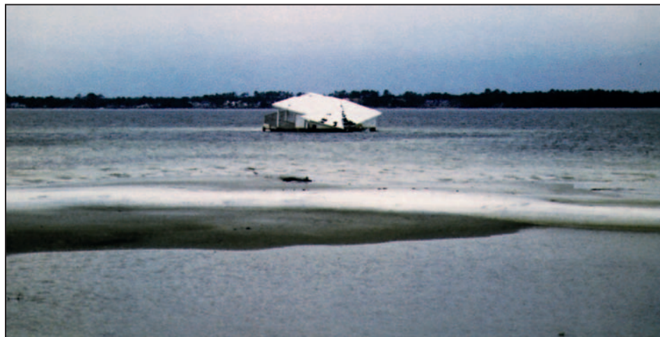
Figure 3-22. This house, located in an area of channeled flow near that shown in Figure 3-20, was undermined, washed into the bay behind the barrier island, and became a threat to navigation
