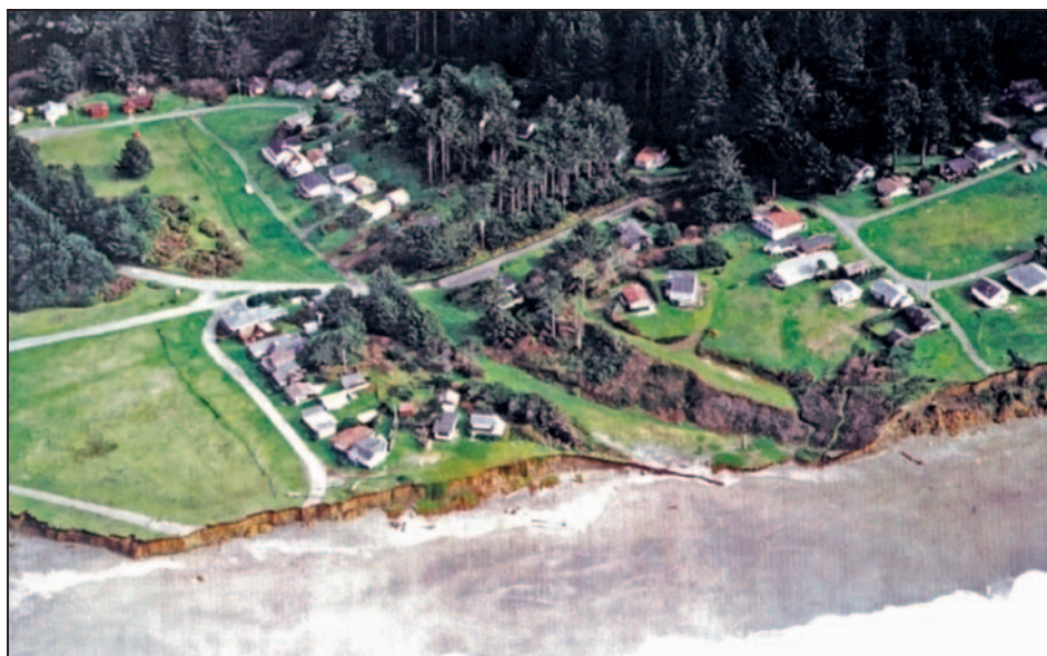
Figure 4-19. As buildings in this Humboldt County, CA, community are threatened by bluff erosion along the Pacific Ocean, they are moved to other sites on the jointly owned parcel
