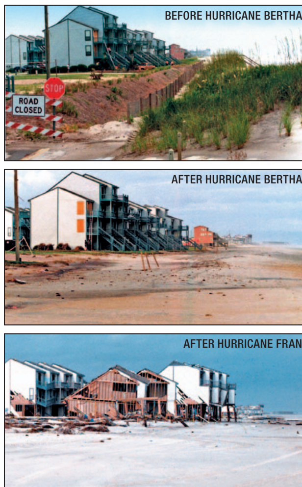
Figure 4-6. Cumulative effects of storms occurring within a short period at one housing development in Jacksonville, NC, July–September 1996
