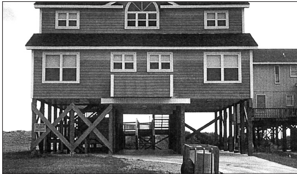
Figure 10-10. Diagonal bracing using dimensional lumber
