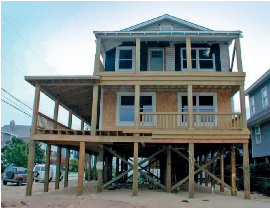
Figure 15-9. Home elevated on piles
