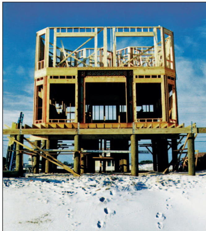
Figure 9-25. Steel moment frame with large opening
