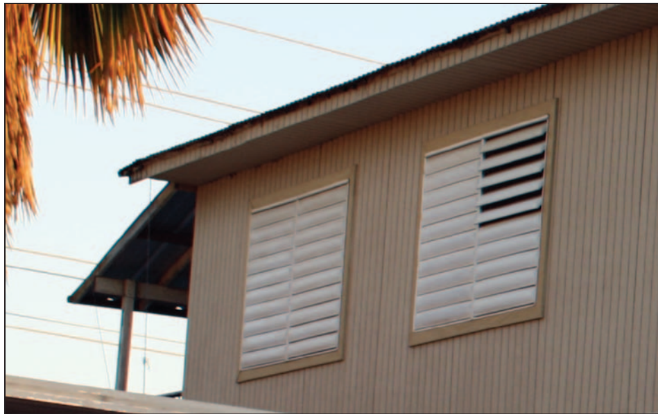
Figure 11-14. House in Puerto Rico with metal jalousie louvers
