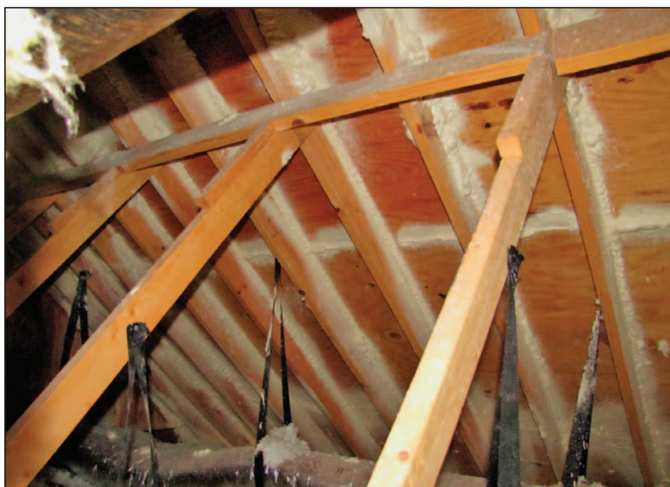
Figure 15-17. Sprayed polyurethane foam adhesive to secure roof deck panels
