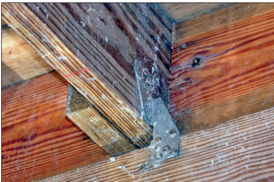
Figure 9-17. Metal joist-to-beam connector
