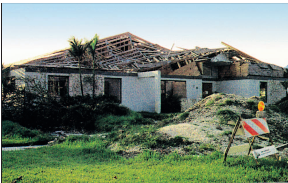
Figure 9-21. Gable-end failure, Hurricane Andrew (Dade County, FL, 1992)
