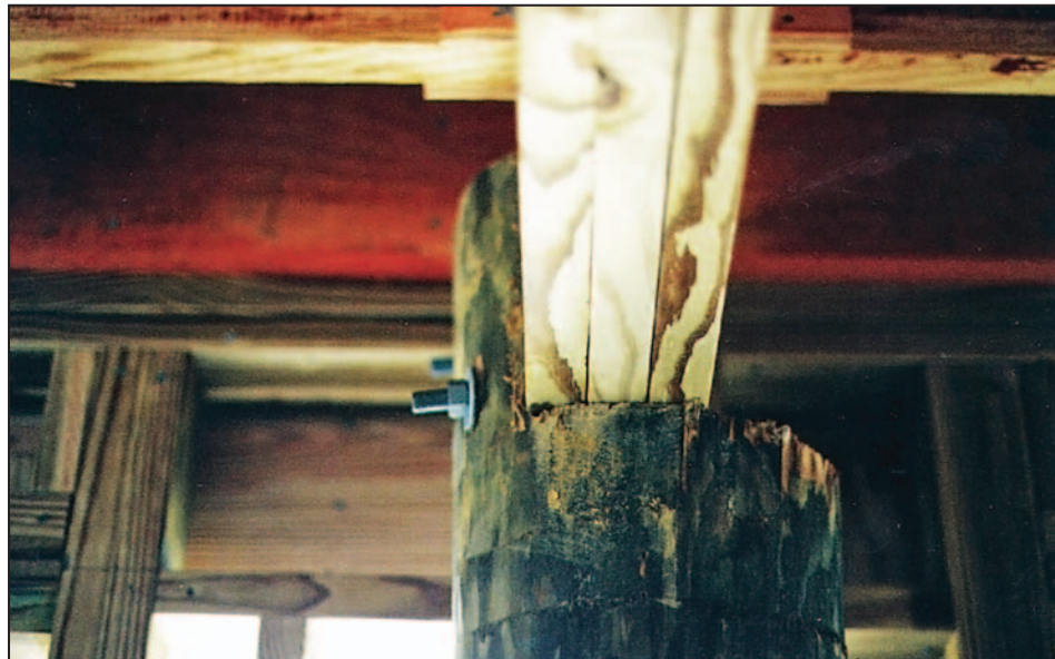
Figure 13-3. Improper overnotched wood pile
