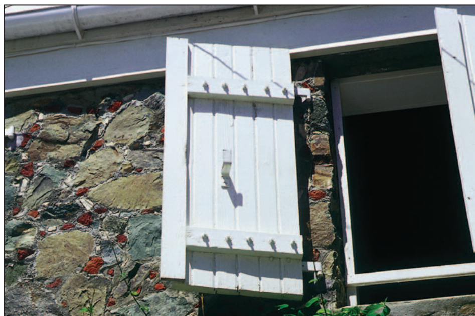
Figure 11-9. Very old building with robust shutters constructed of 2x4 lumber, bolted connections, and heavy metal hinges. Hurricane Marilyn (U.S. Virgin Islands, 1995)
