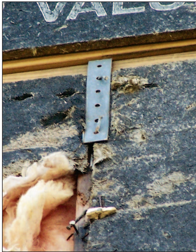
Figure 13-15. Connector failure caused by insufficient nailing
