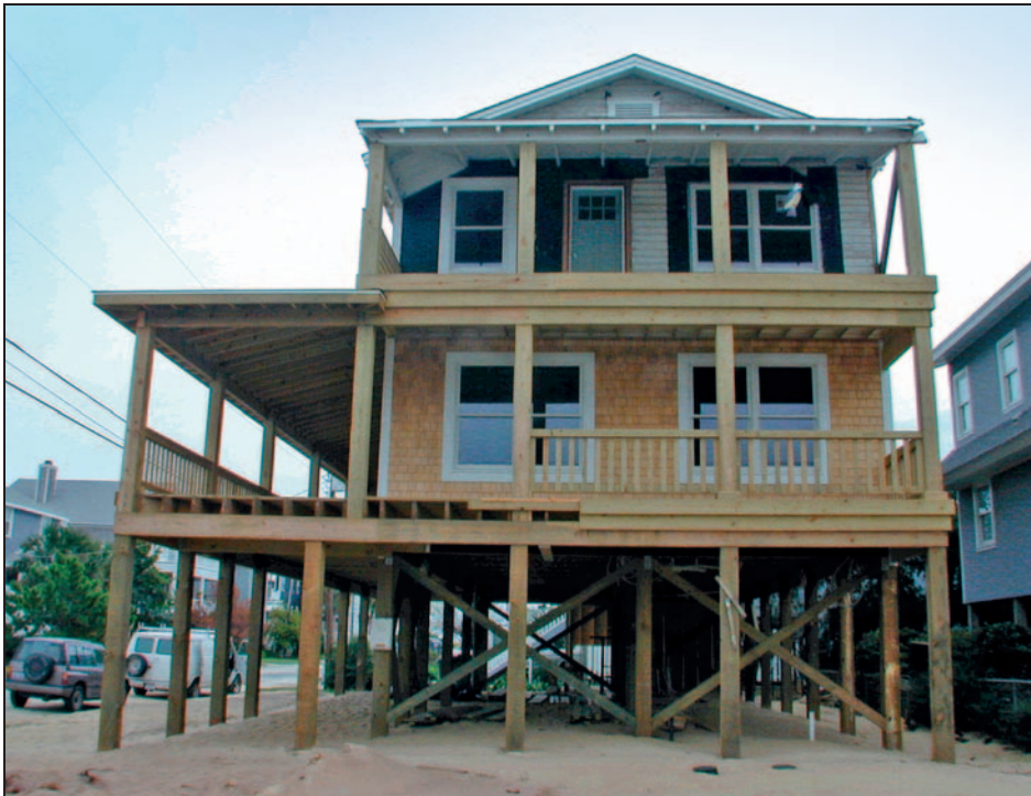
Figure 15-9. Home elevated on piles
