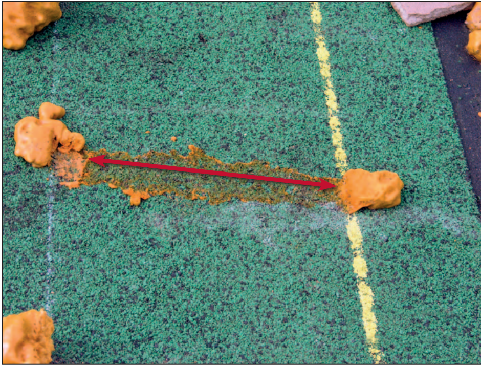
Figure 11-44. Adhesive that debonded from the cap sheet
