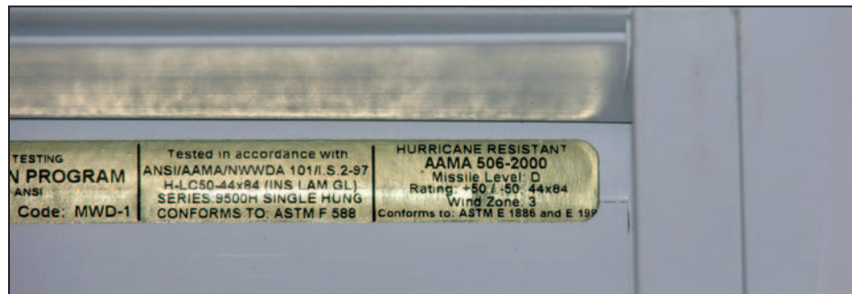
Figure 11-11. Design pressure and impact-resistance information in a permanent window label. Hurricane Ike (Texas, 2008)
