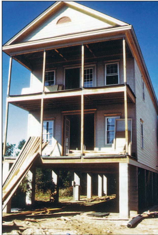
Figure 13-6. Open masonry foundation
