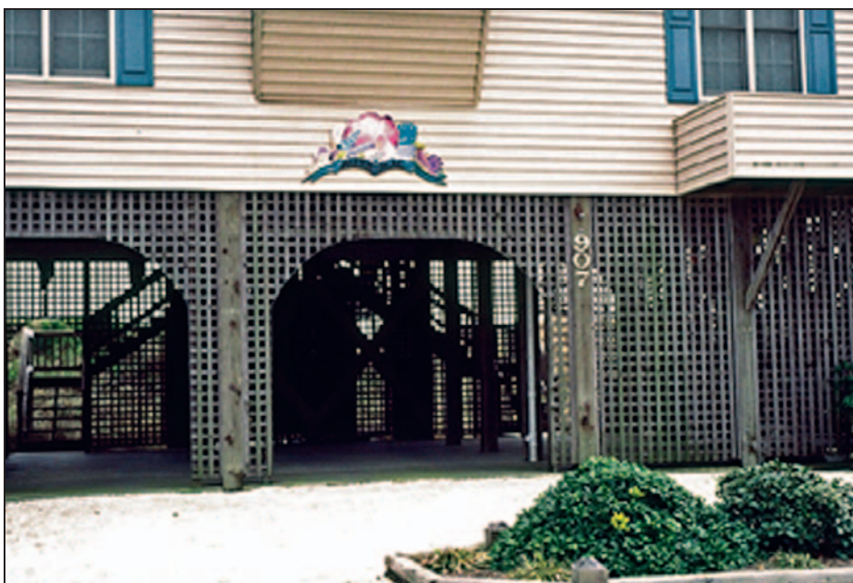
Figure 9-30. Lattice beneath an elevated house in Zone V
