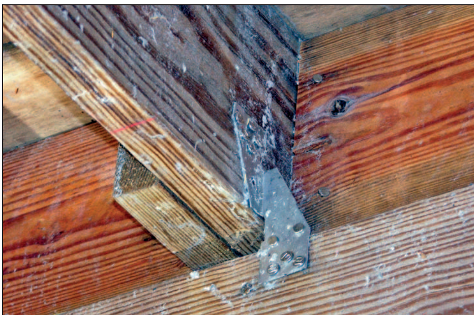
Figure 9-17. Metal joist-to-beam connector
