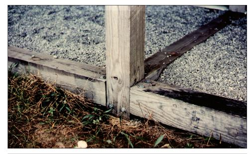
Figure 2-4. Near collapse due to insufficient pile embedment (Dauphin Island, Alabama).
