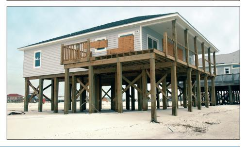
When used with grade beams, the piles and grade beams work in conjunction to elevate the structure, provide vertical and lateral support for the elevated home, and transfer loads imposed on the elevated home and foundation to the ground below.
