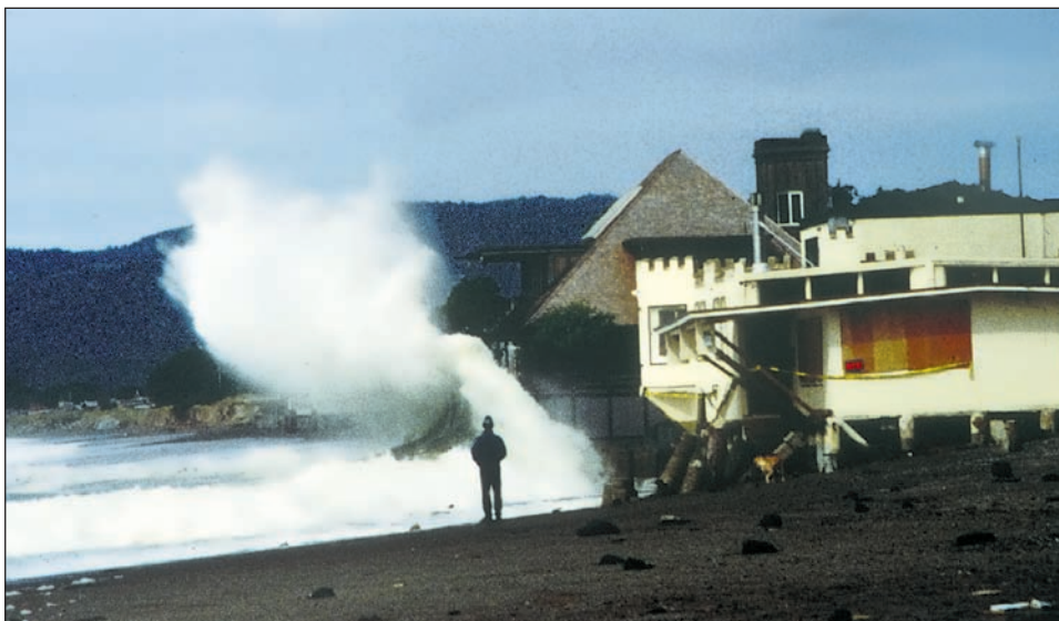
Figure 1-10. Storm waves breaking against a seawall in front of a coastal residence at Stinson Beach, California.
