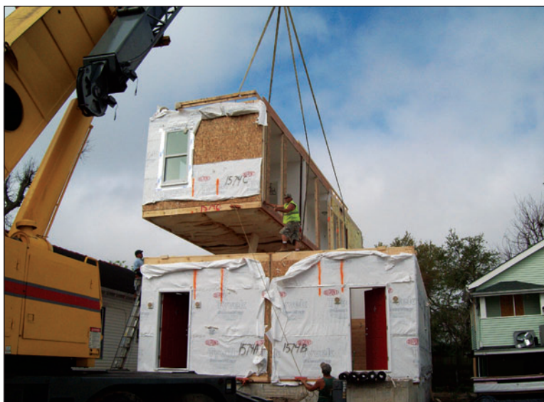
Figure 1. Construction of a modular home.
