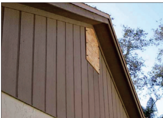
Figure 10. Shuttered gable end vent.
