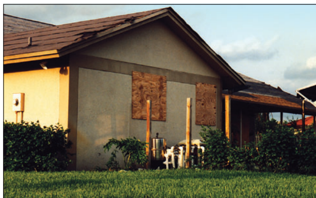
Figure 1. Wood structural panels installed in accordance with building code requirements are a cost-effective means of protection, but they should be adequately attached so they themselves do not become windborne debris.
