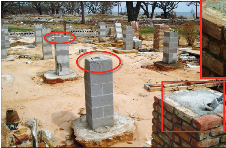
Figure 3. Failure of pier-to-beam connections due to wave and flood forces acting on the elevated building (Long Beach, Mississippi)
