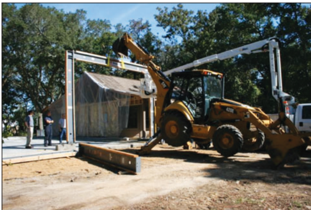
Figure 4. Installation of a prefabricated ordinary moment frame.
