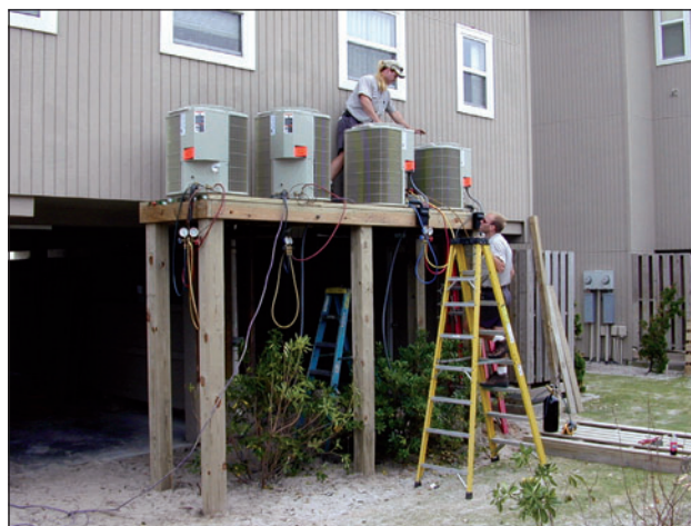
Elevated air conditioning compressors.
