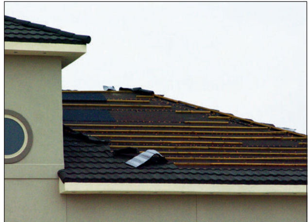
Figure 7. This residence had metal shingles that simulated the appearance of tile. The shingles typically blew off the battens, but some of the battens were also blown away.
