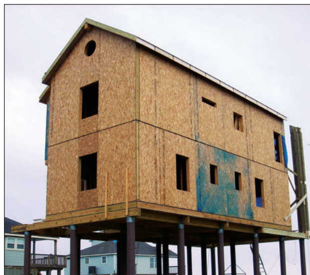
Figure 2. Construction of a Structural Insulated Panel house.
