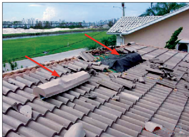
Figure 11. Two off-ridge vents are shown in this photograph. The vent that is covered with roofing felt flipped up and allowed a substantial amount of water to enter the residence. Carpeting, kitchen cabinets, and a large amount of gypsum board had to be replaced because of the water intrusion.
