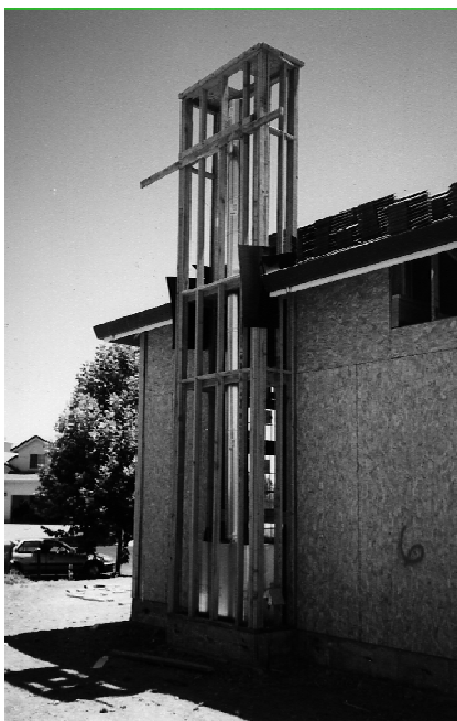
Figure 7-7 Factory-built flue and light-frame enclosure.
