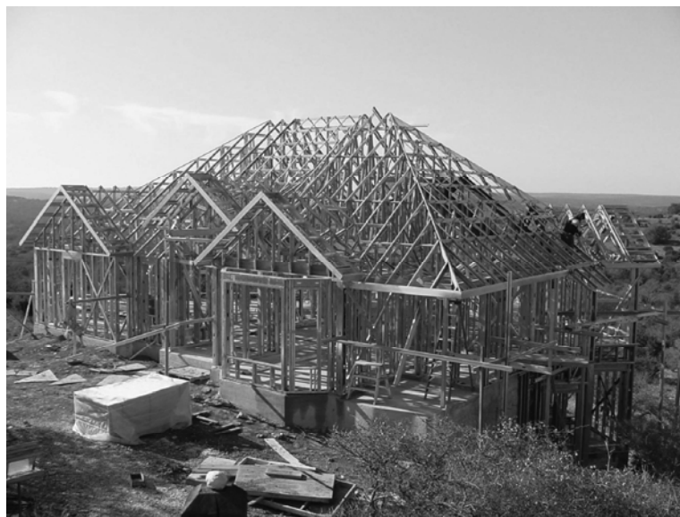
Figure 5-13 Cold-formed steel house under construction. Photo Courtesy of Dietrich Metal Framing -- a Worthington Industries Company
