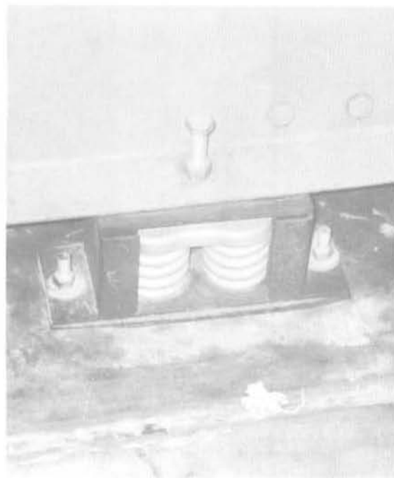
Chiller mount with no uplift resistance and insufficient or no shear resistance. Photo Credit: Wiss, Janney, Elstner Associates, Inc.
