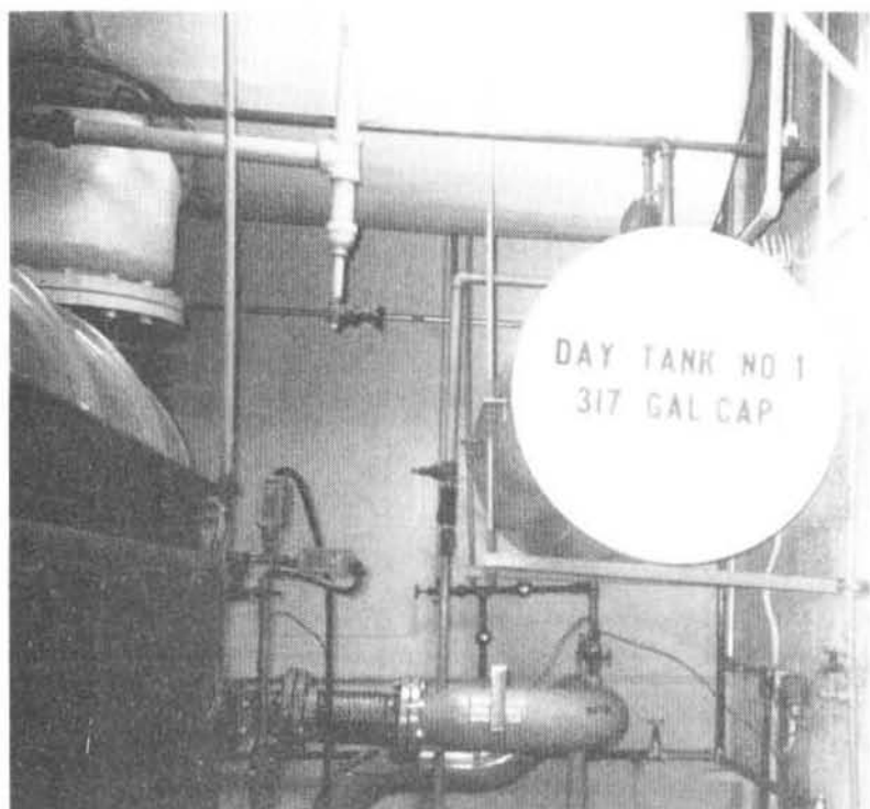
Unbraced Day Tank, Hospital, Puerto Rico
