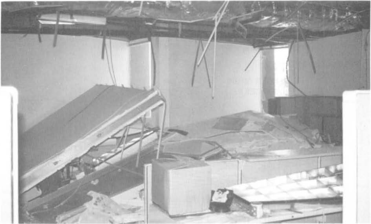
Failure of office partitions, ceilings, and light fixtures Earthquake Damage: 1994, Northridge, California Photo Credit: Wiss, Janney, Elstner Associates, Inc.
