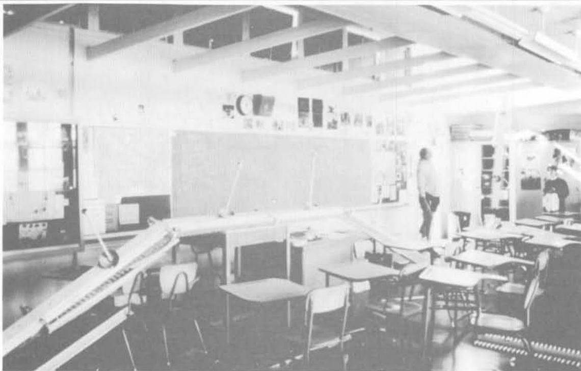
Failure of light fixtures at Northridge Junior High School
