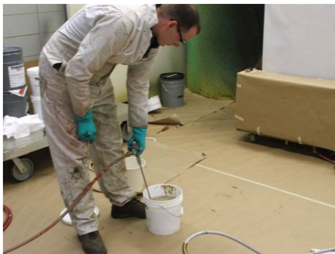
FIGURE A-4. Pre-mix of the elastomeric coating components.
