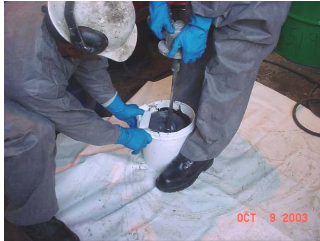
FIGURE A-9. Mixing a kit of sealing/fairing compound.
