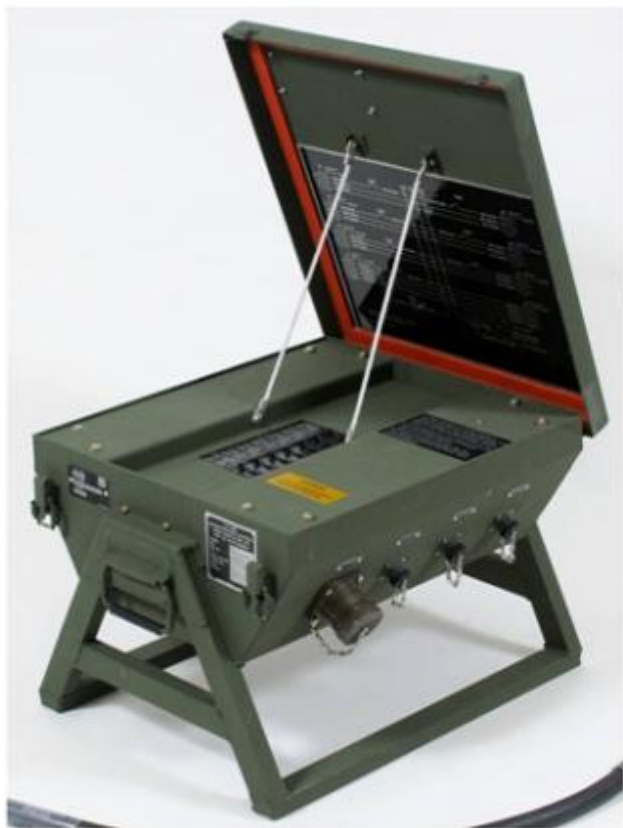
FIGURE B- 7 PDISE, M60 Electrical Distribution System
