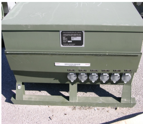
FIGURE B- 26 150KW, 30KVA Power Distribution Panel
